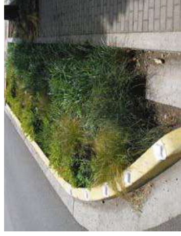
Above: An example curb that supports stormwater retention and groundwater infiltration.
