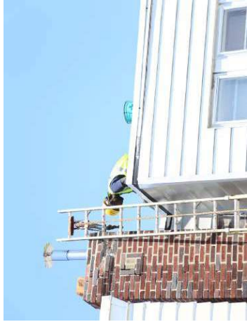
Above: Roof repairs on a Philadelphia home as part of the Basic Systems Repair Program.
