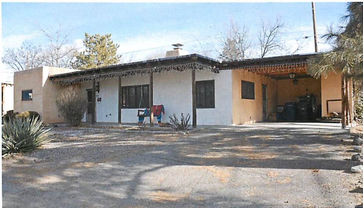
Photo 1: Street and south elevations, facing southeast.
