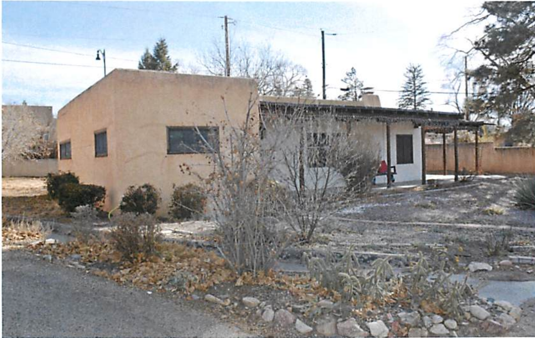
Photo 2: Street and north elevations, facing southeast.
