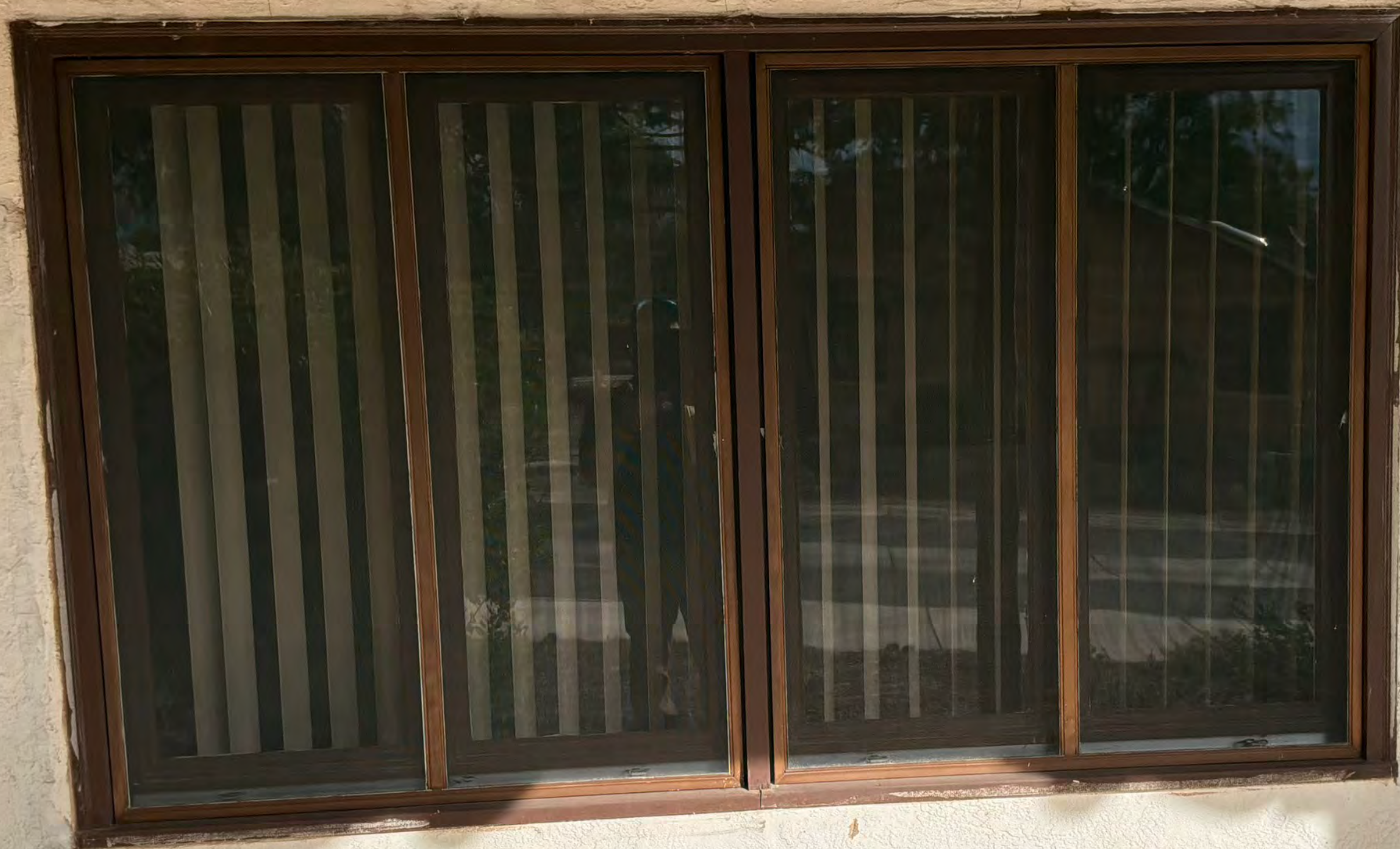
West Elevation Window B.
