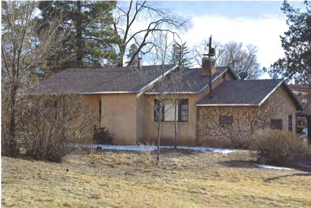
Photo 3: North elevation, facing southeast.
