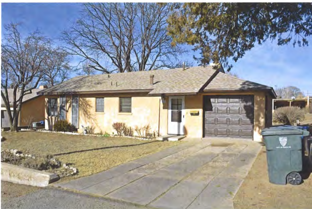
Photo 2: Street and east elevations, facing northeast.
