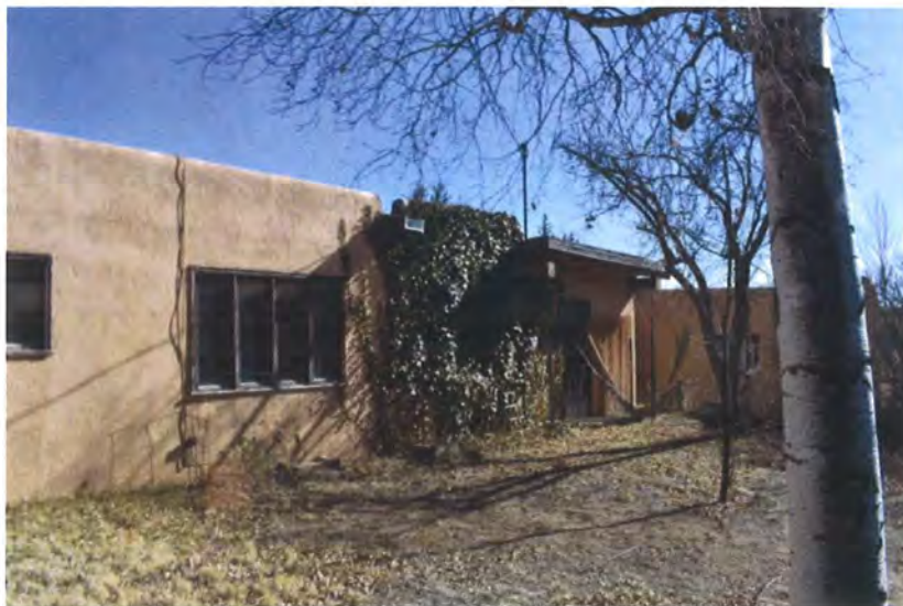
Photo 2: West elevation, facing southwest (Sharon Joyce, February 23, 2018).
