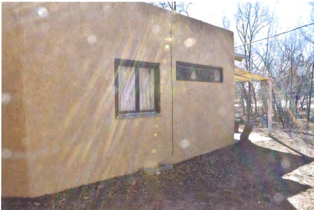
Photo 3: North elevation, facing southwest (Sharon Joyce, February 23, 2018).
