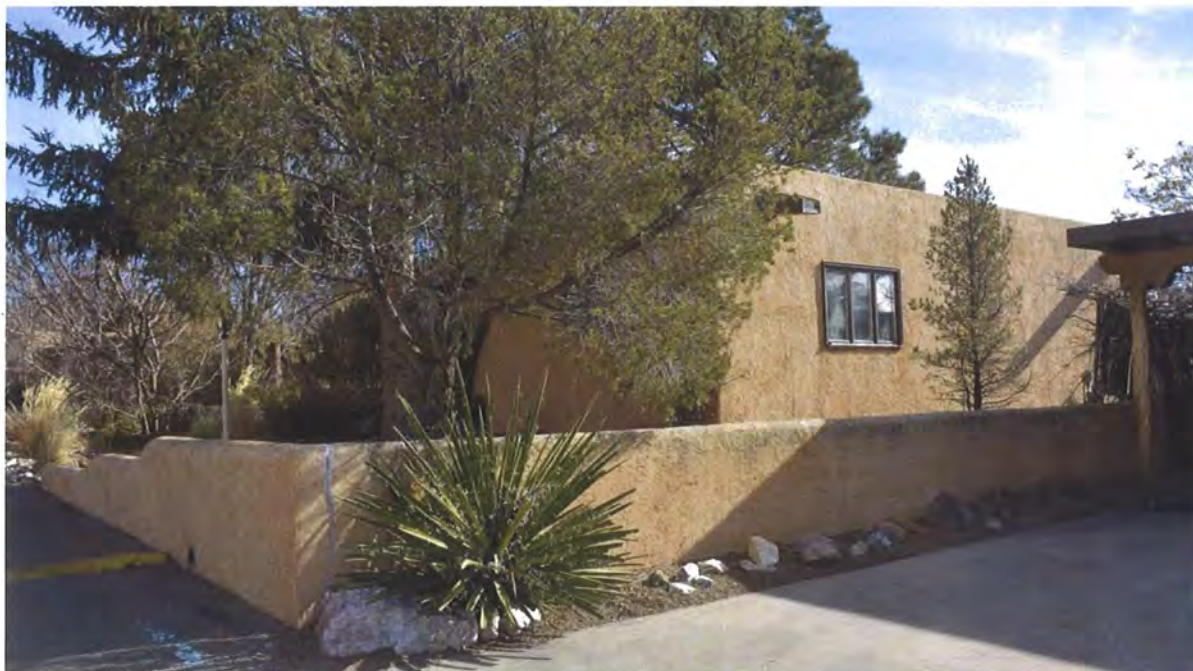
Photo 2: West elevation, facing southeast.
