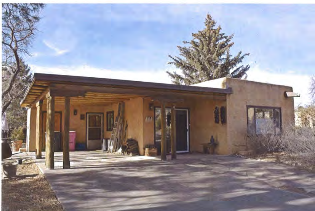
Photo 1: East and south elevations, facing northeast.
