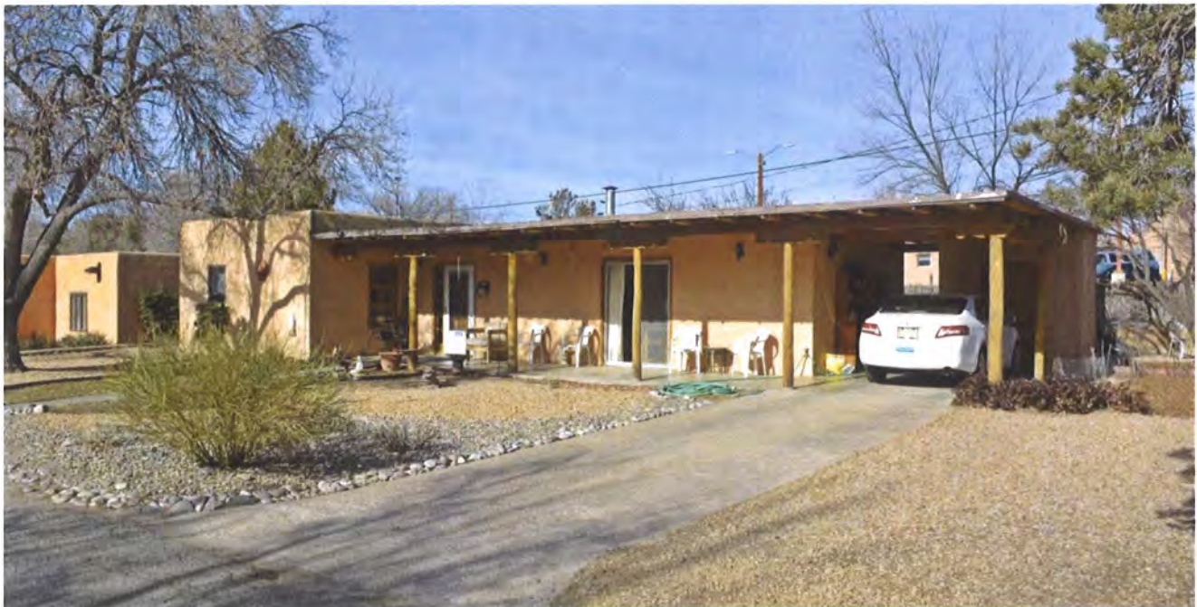
Photo 1: Street and east elevations, facing northwest.
