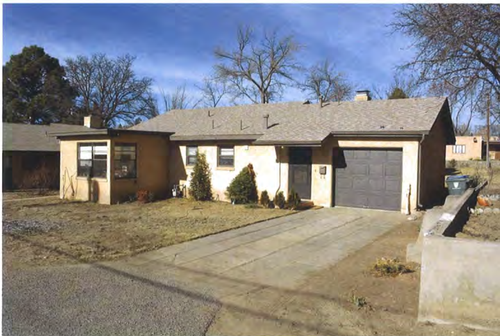
Photo 1: Street and east elevations, facing northwest.
