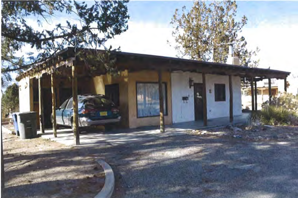
Photo 2: South and east elevations, facing northwest.
