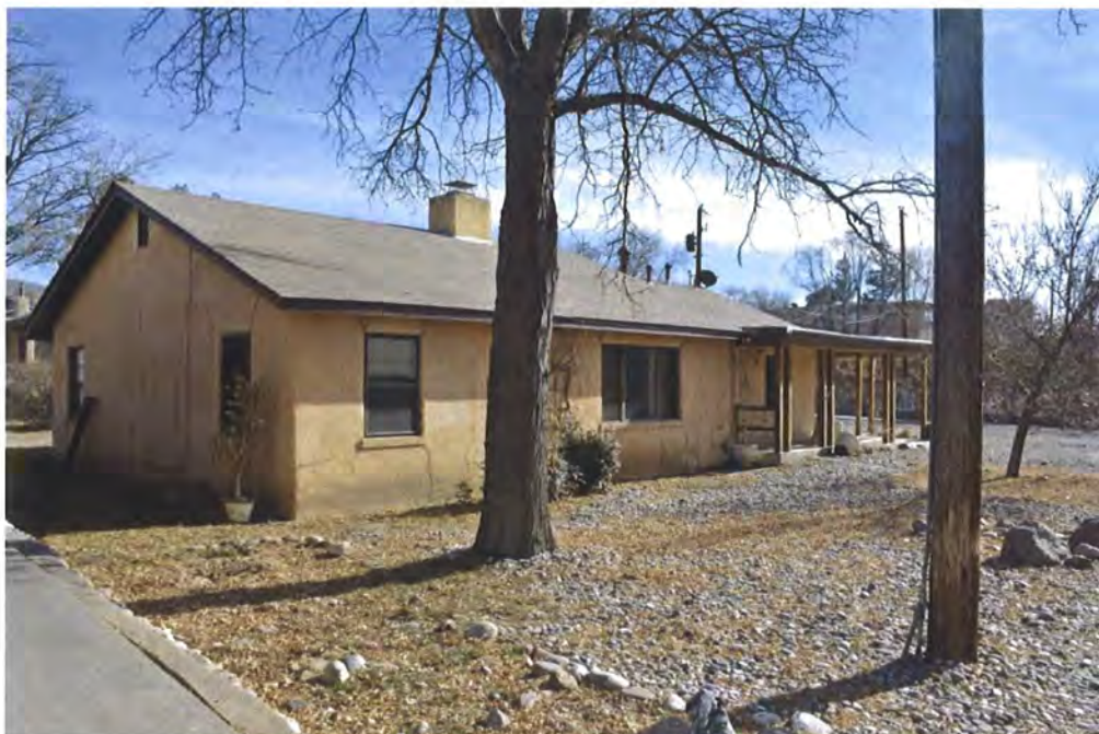
Photo 2: North and west elevations, facing southeast.
