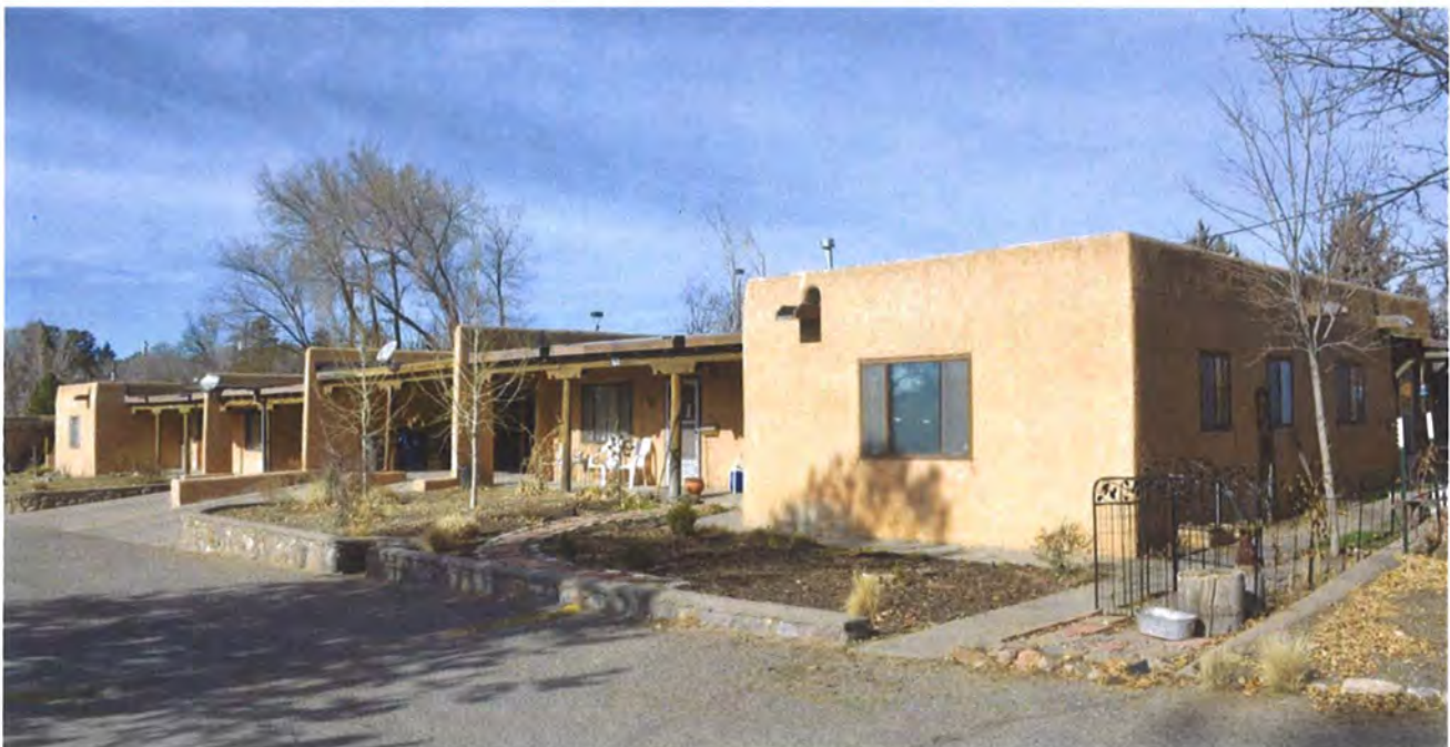
Photo 1: Street elevation and east elevations, facing northwest.
