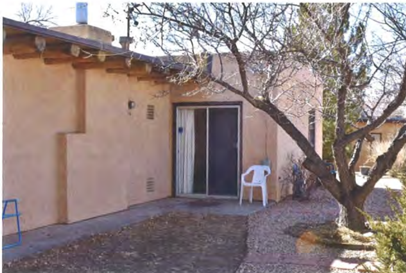
Photo 3: North elevation, facing southwest (Sharon Joyce, February 23, 2018).
