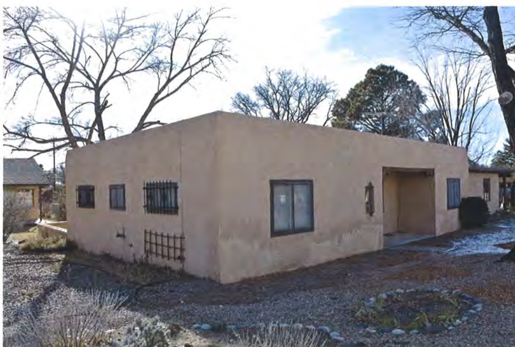
Photo 1: Street and north elevations, facing southeast.
