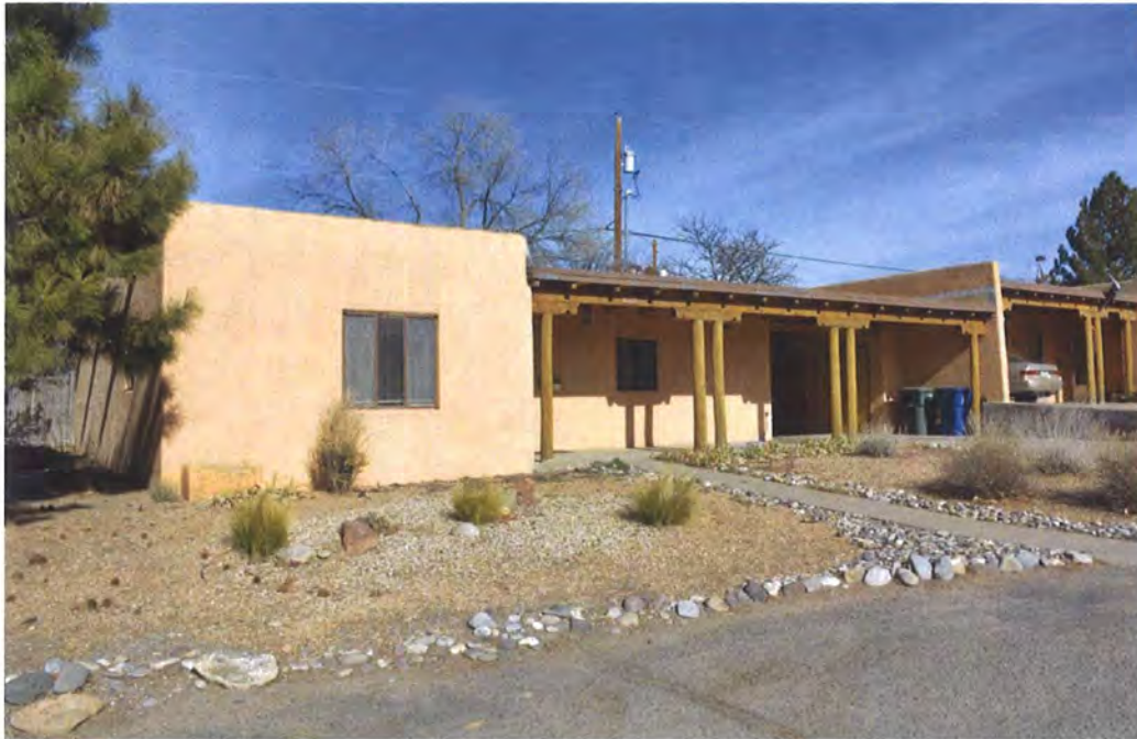
Photo 2: Street and west elevations, facing northeast.
