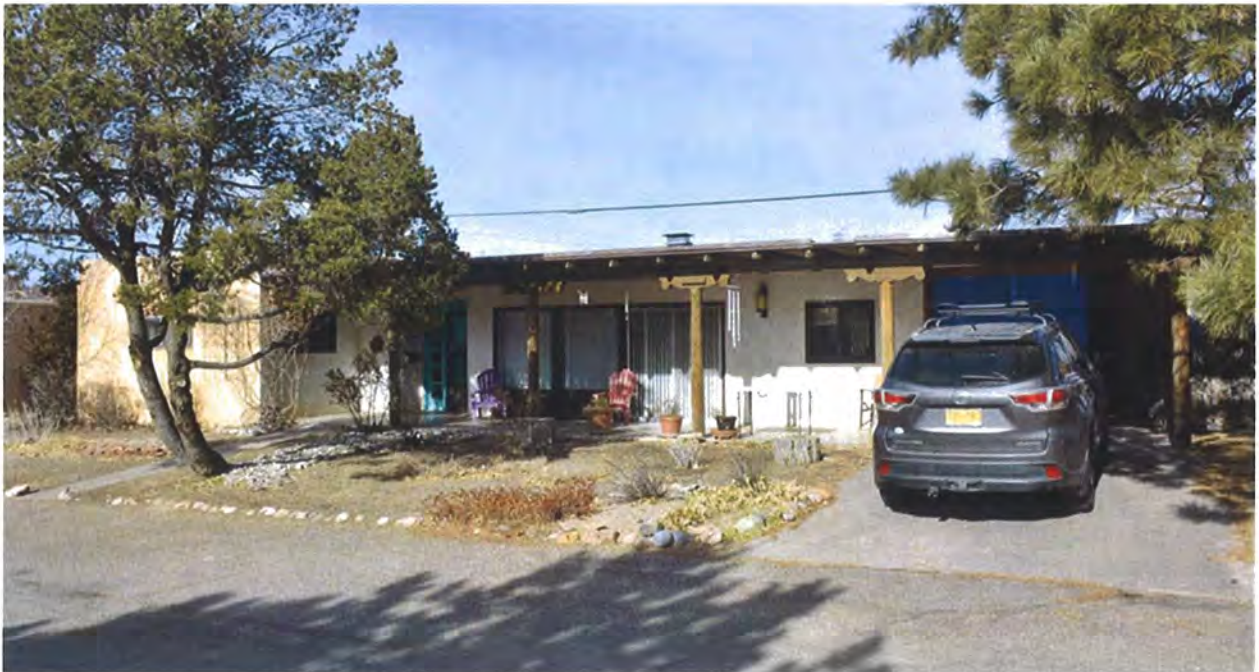
Photo 1: Street and east elevations, facing northwest.
