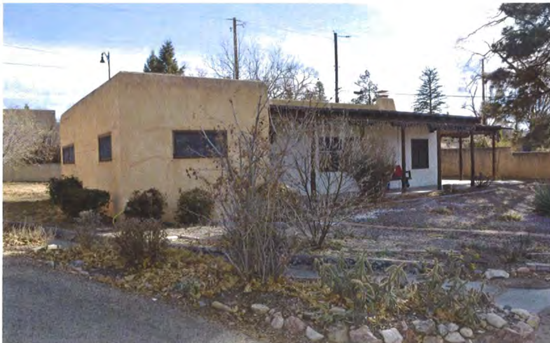
Photo 2: Street and north elevations, facing southeast.
