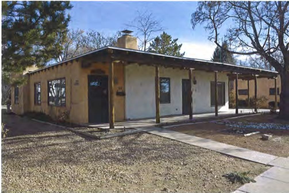
Photo 2: North and street elevations, facing southeast.
