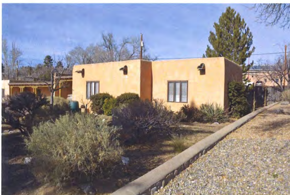
Photo 1: Street and east elevations, facing northwest.
