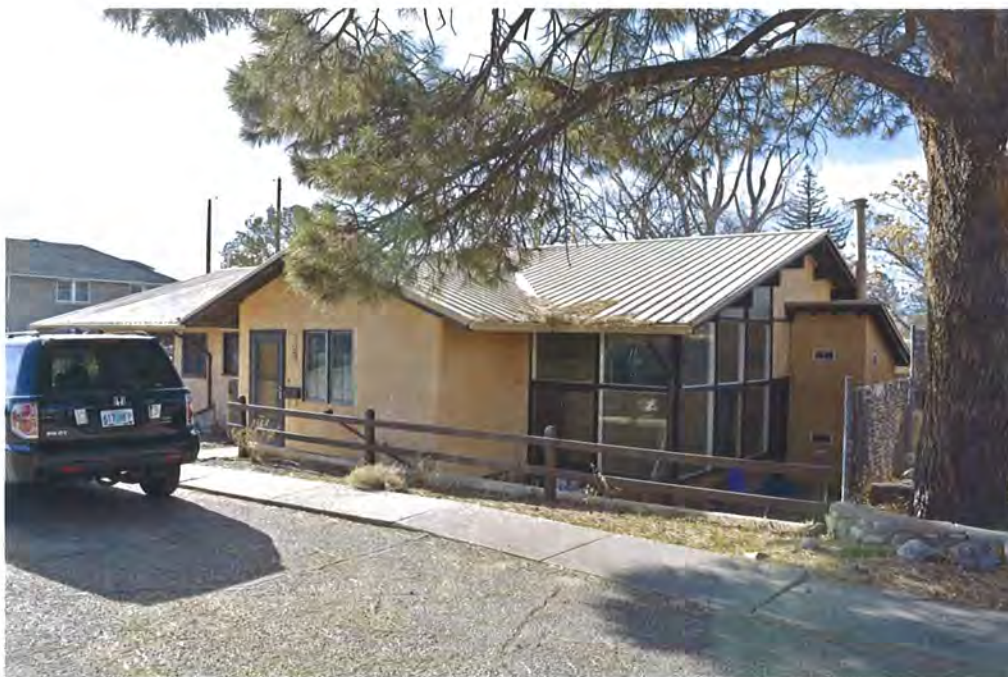
Photo 1: Street and north elevations, facing southwest.
