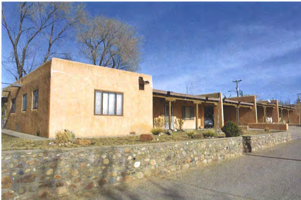
Photo 2: Street and west elevations, facing northeast.
