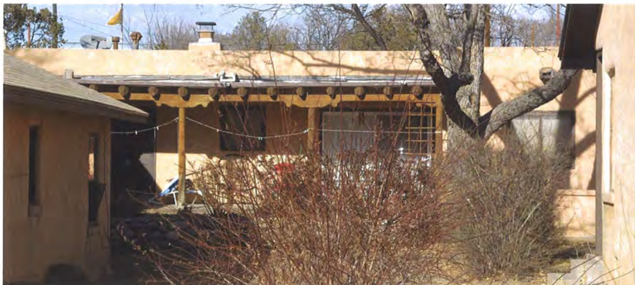
Photo 4: South elevation, facing north.
