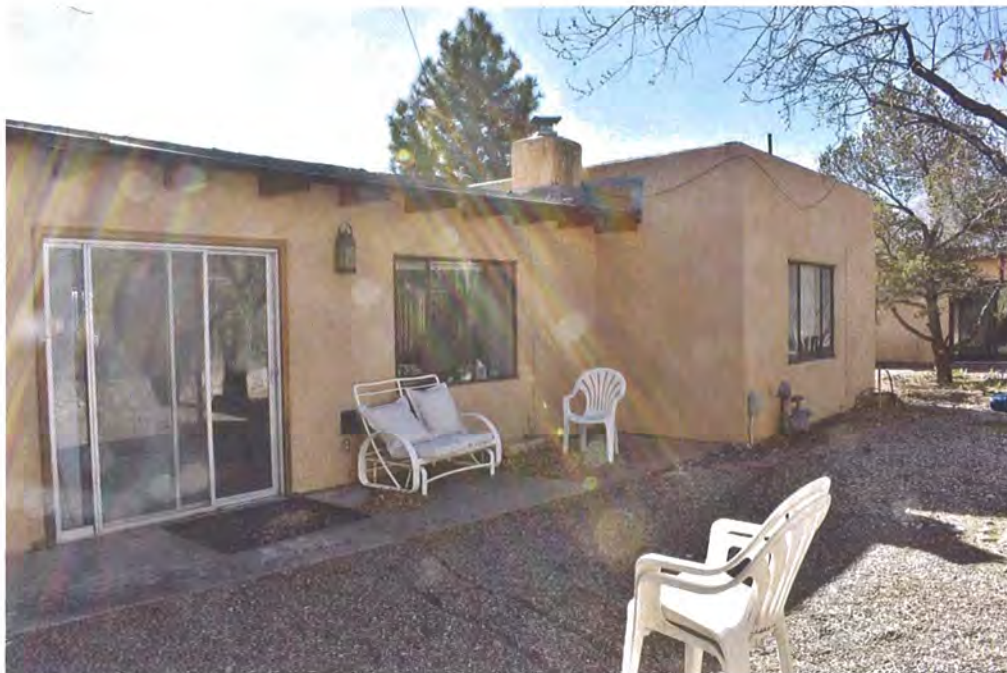
Photo 3: North elevation, facing southwest (Sharon Joyce, February 23, 2018).
