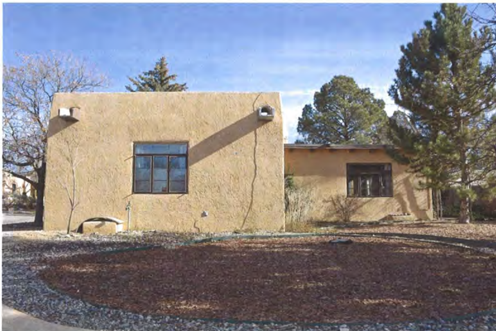
Photo 2: West elevation, facing east.
