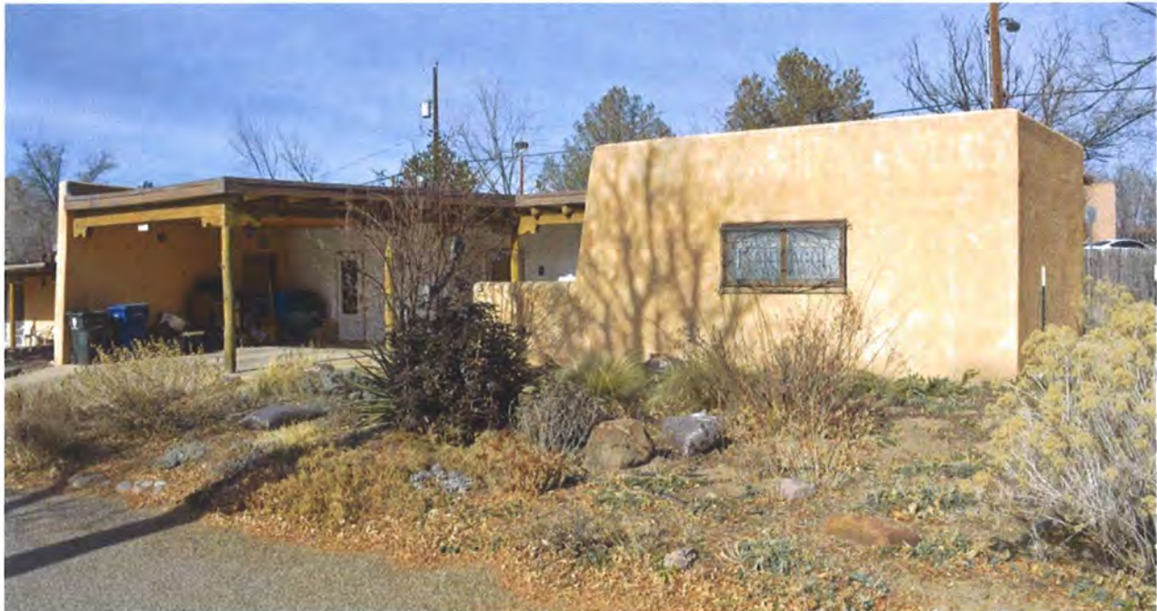
Photo 1: Street and east elevations, facing northwest.
