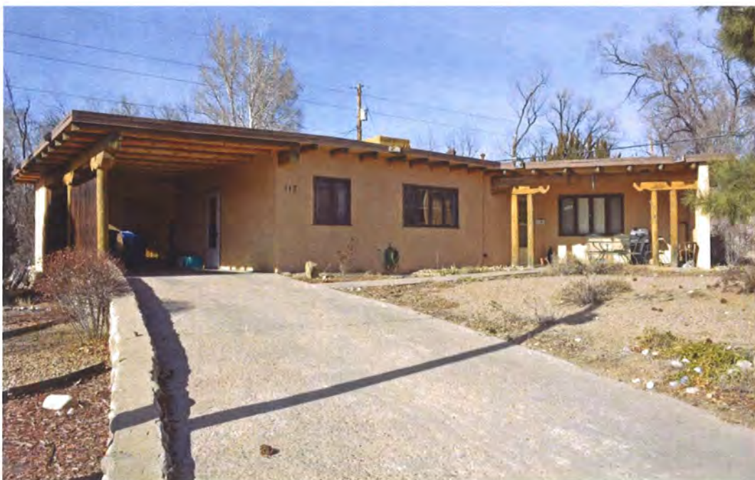
Photo 1: Street, west and south elevations, facing northeast.
