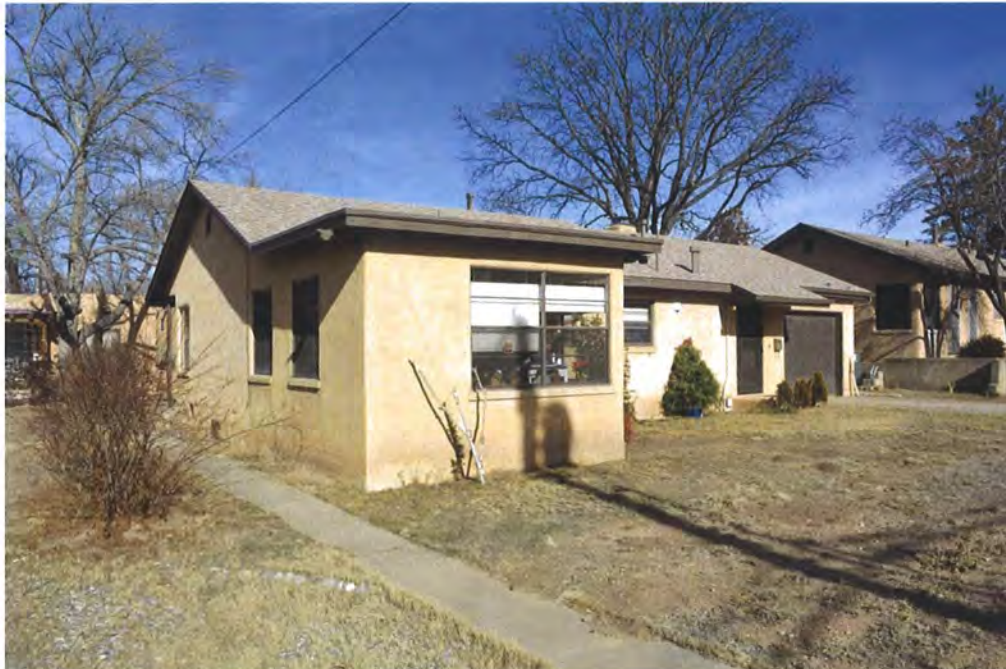
Photo 2: Street and west elevations, facing northeast.
