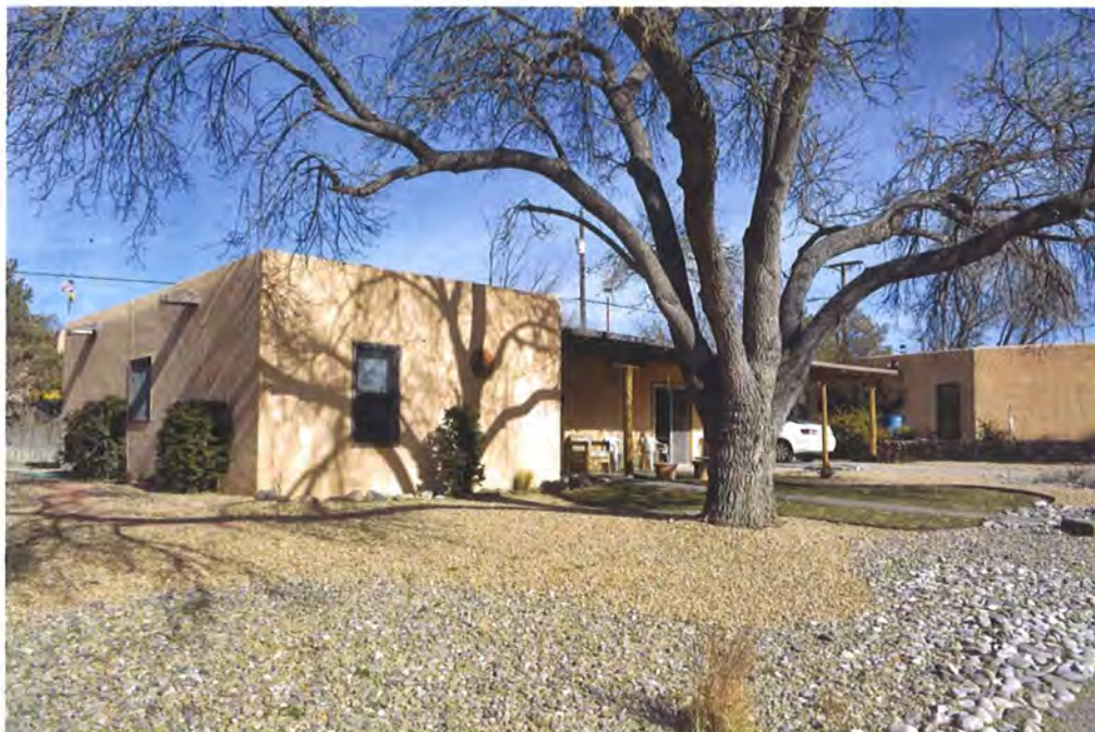
Photo 2: Street and west elevations, facing northeast.
