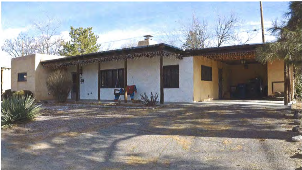
Photo 1: Street and south elevations, facing southeast.
