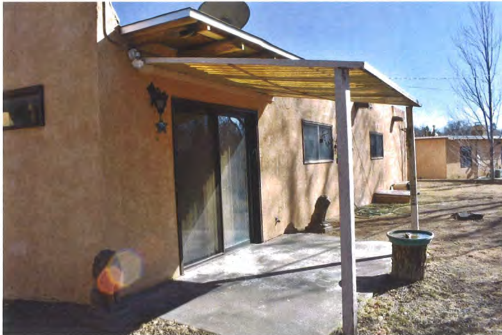
Photo 2: West elevation, facing south (Sharon Joyce, February 23, 2018).
