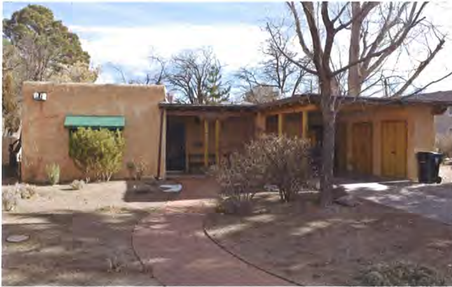
Figure 12: 120 Camino Santiago, constructed in c. 1971.
