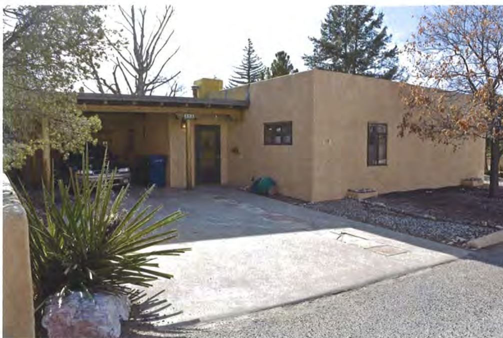
Photo 1: Street and east elevations, facing southwest.
