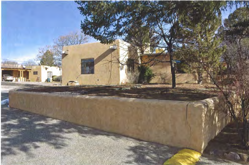
Photo 3: West and south elevations, facing northeast.
