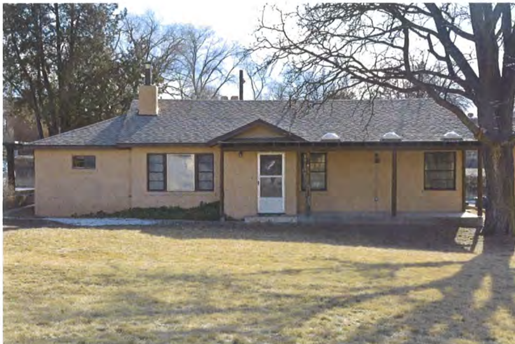
Photo 2: North elevation, facing south.
