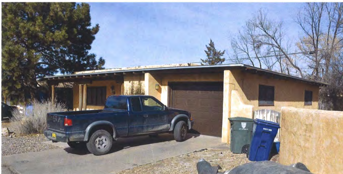
Photo 1: Street elevation and north elevations, facing northwest.
