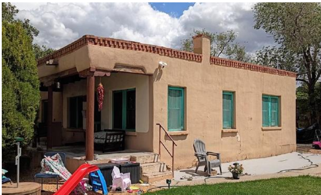
Figure 2: The Residence Northwest Corner
