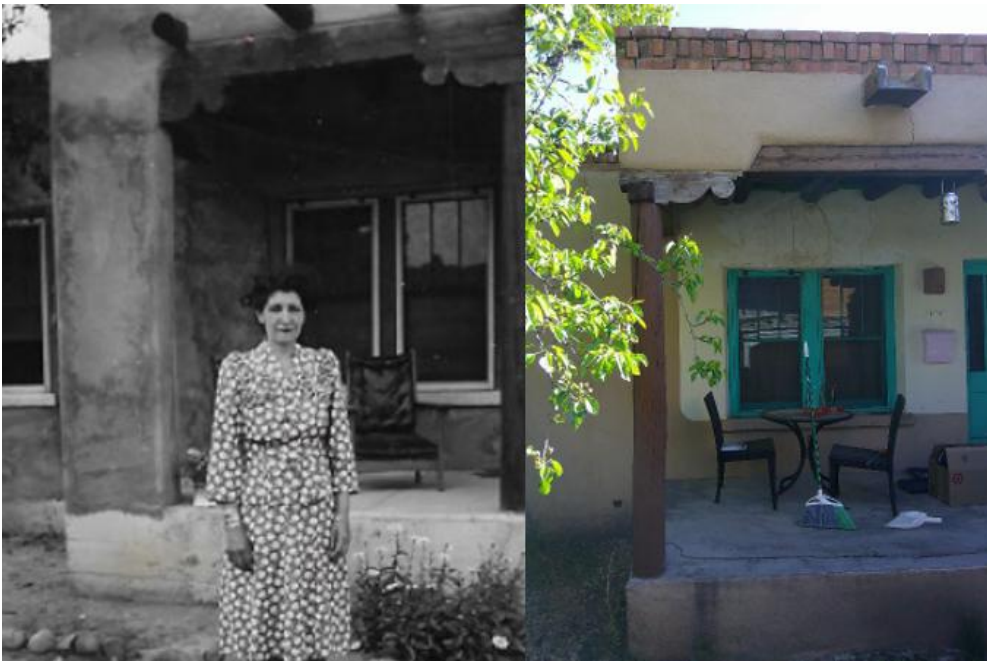
Figure 3: Portal Columns 1930s and 2026
