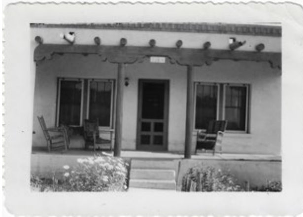
Original North Façade, circa early 1940's
