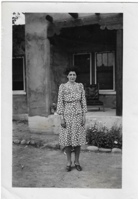
North Façade Entry Portal after stucco work circa 1930's Ruby Gonzales Chapman
