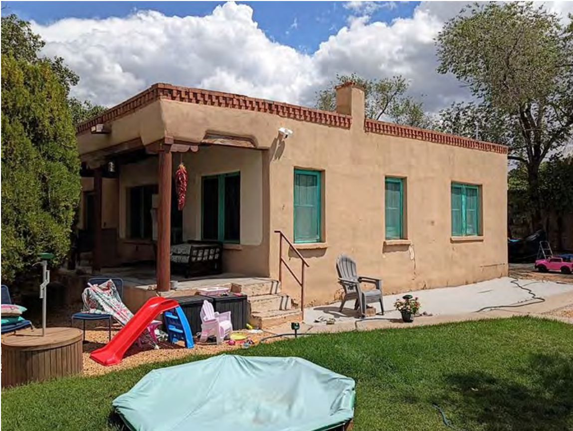
Photo 8: West elevation. Camera facing southeast.
