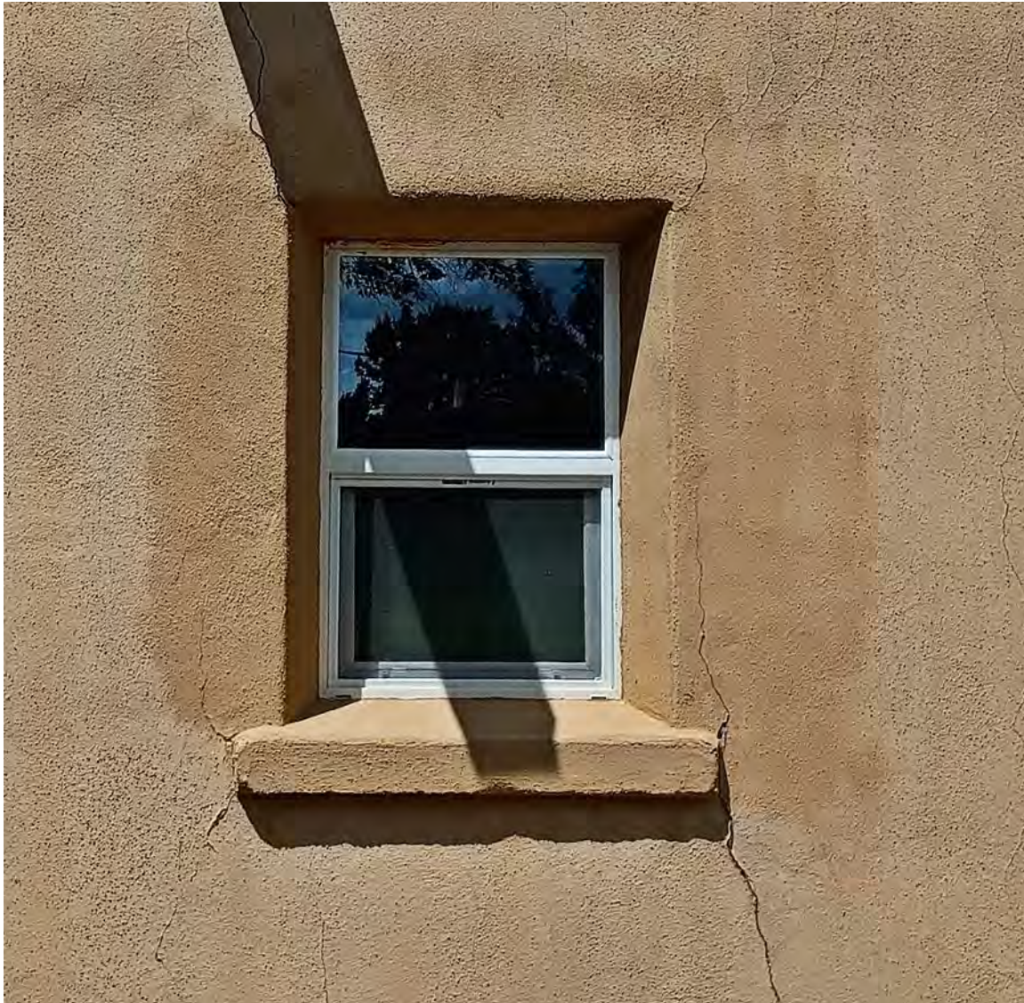
Photo 10: South elevation. Detail of replacement window.
