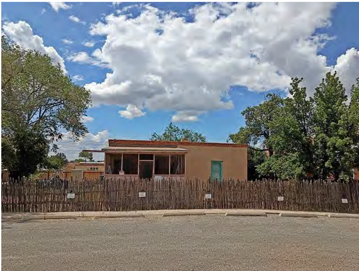
Photo 2: Setting from leased parking lot. Camera facing west.
