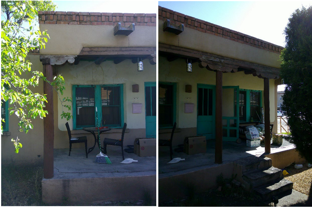
North Façade Entry Portal
