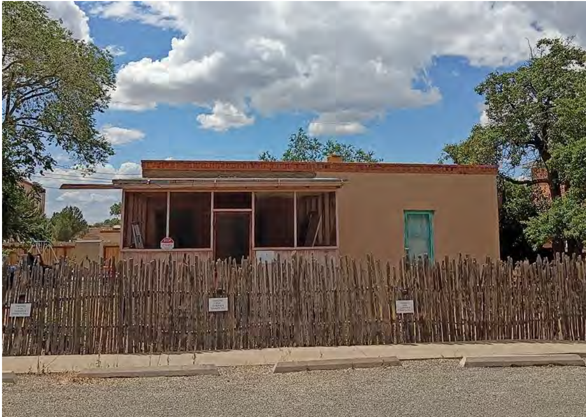
Photo 12: East elevation. Camera facing west.
