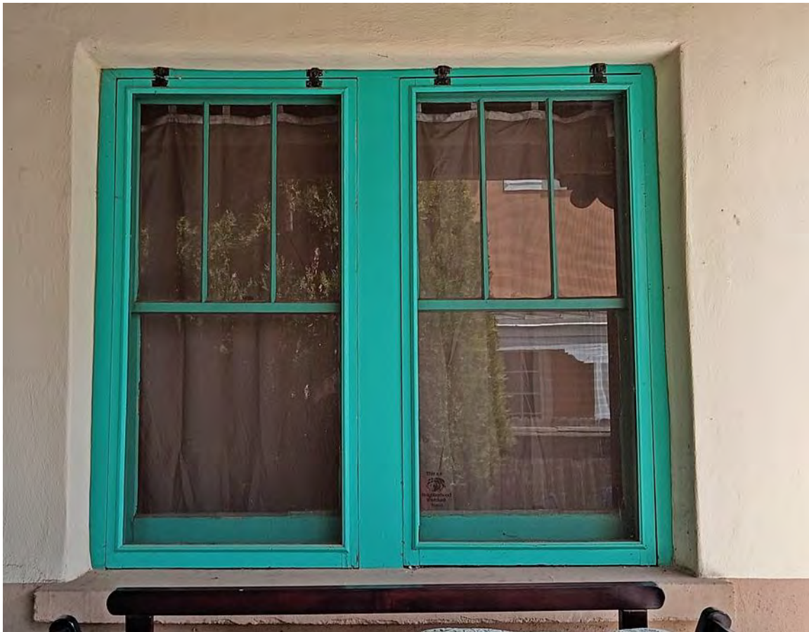
Photo 7: North elevation. Window detail. Camera facing south.
