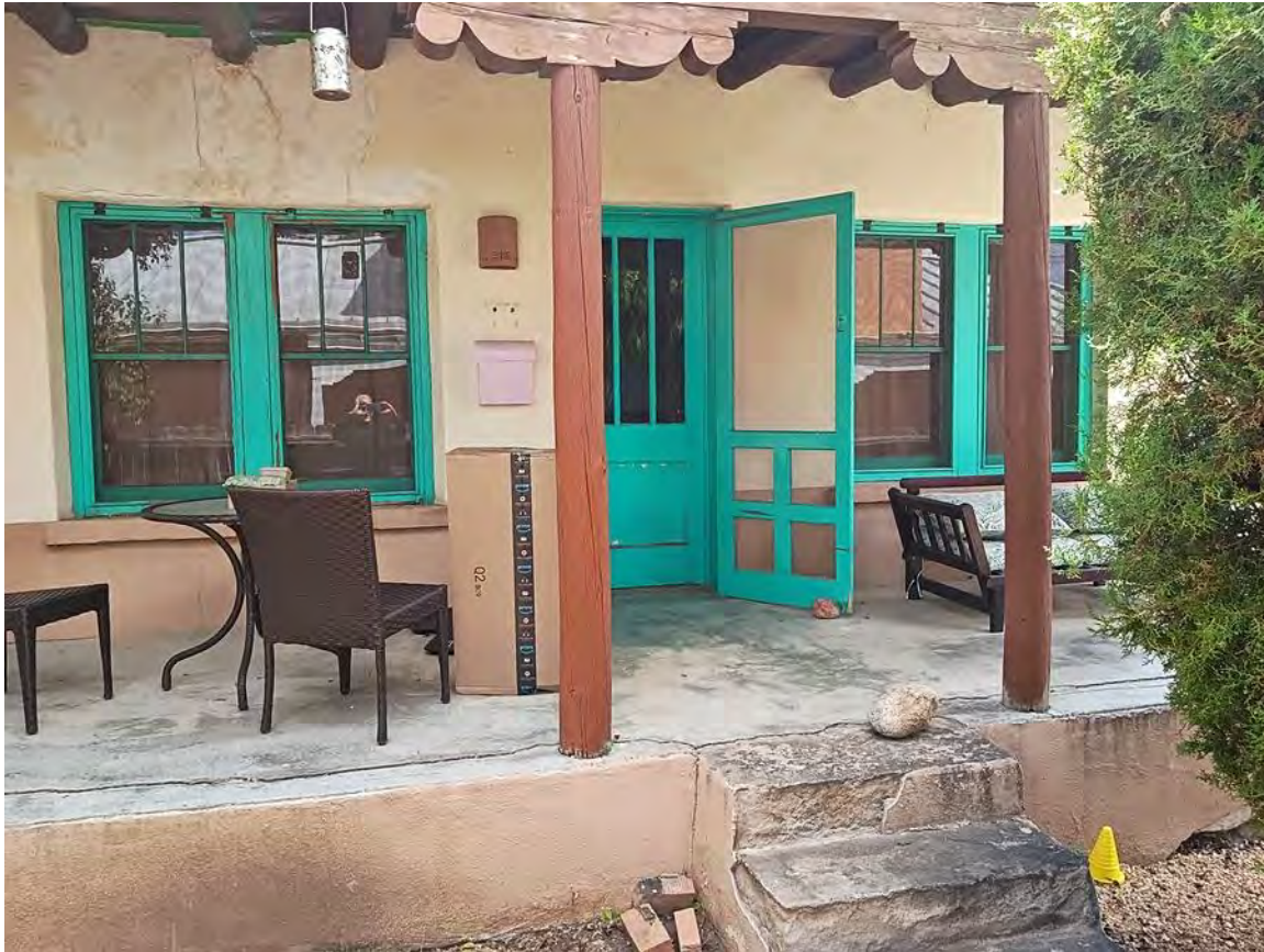
Photo 6: North elevation. Camera facing southwest.
