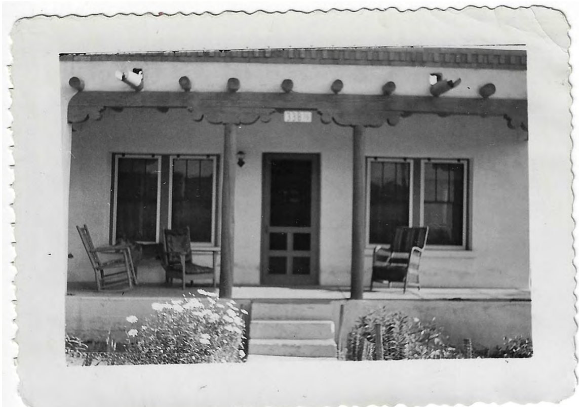
Figure 3: Undated photograph. Note presence of viga ends and rounded galvanized canales. Courtesy of the Alarid family.
