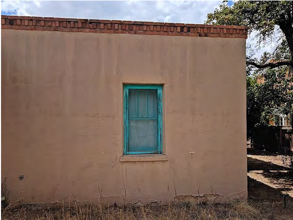
Photo 13: East elevation, north end. Camera facing northwest.
