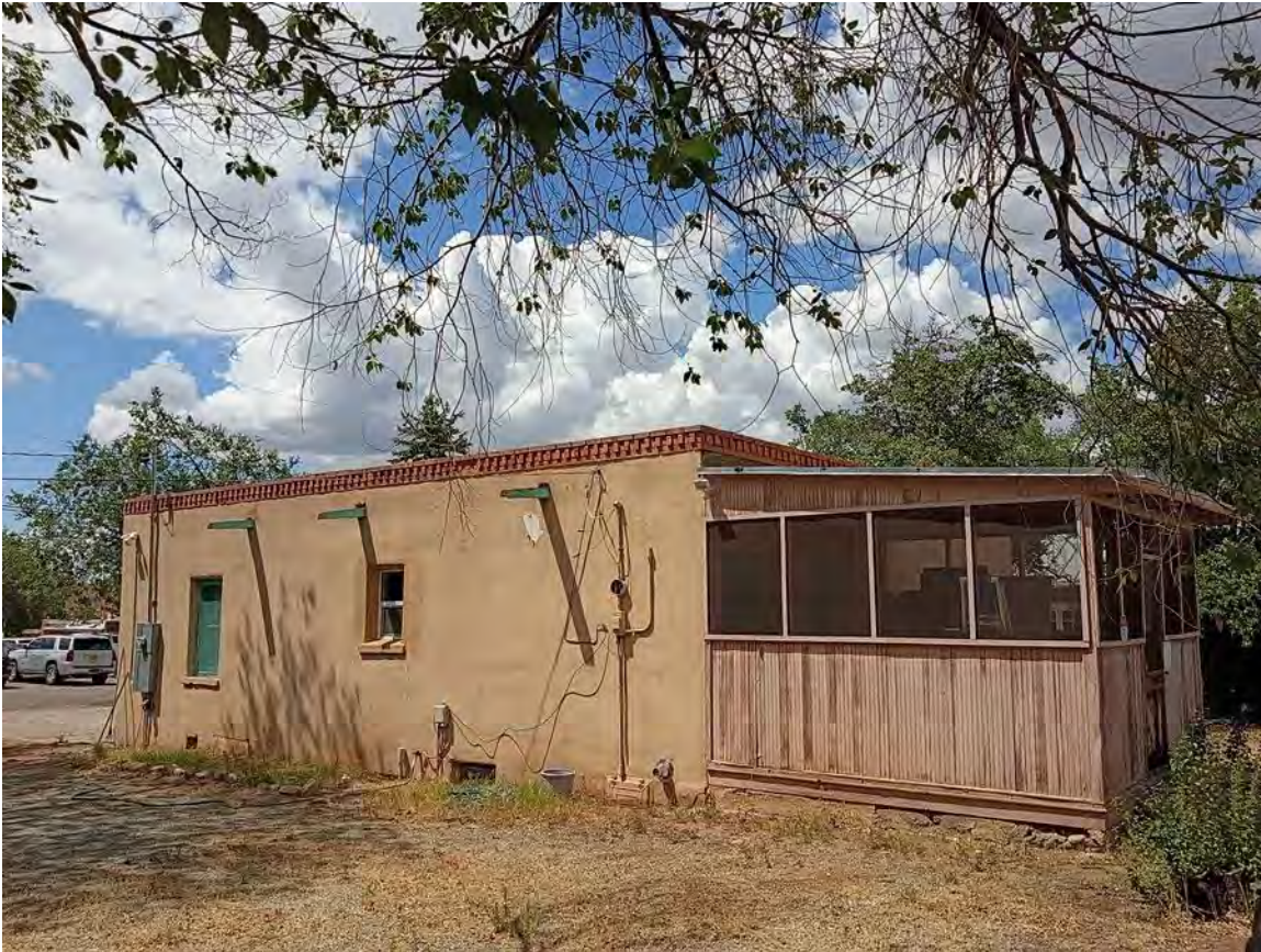
Photo 9: South elevation. Camera facing northwest.
