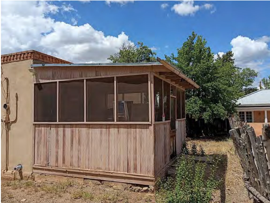
Photo 11: South elevation. Frame screen porch. Camera facing northwest.
