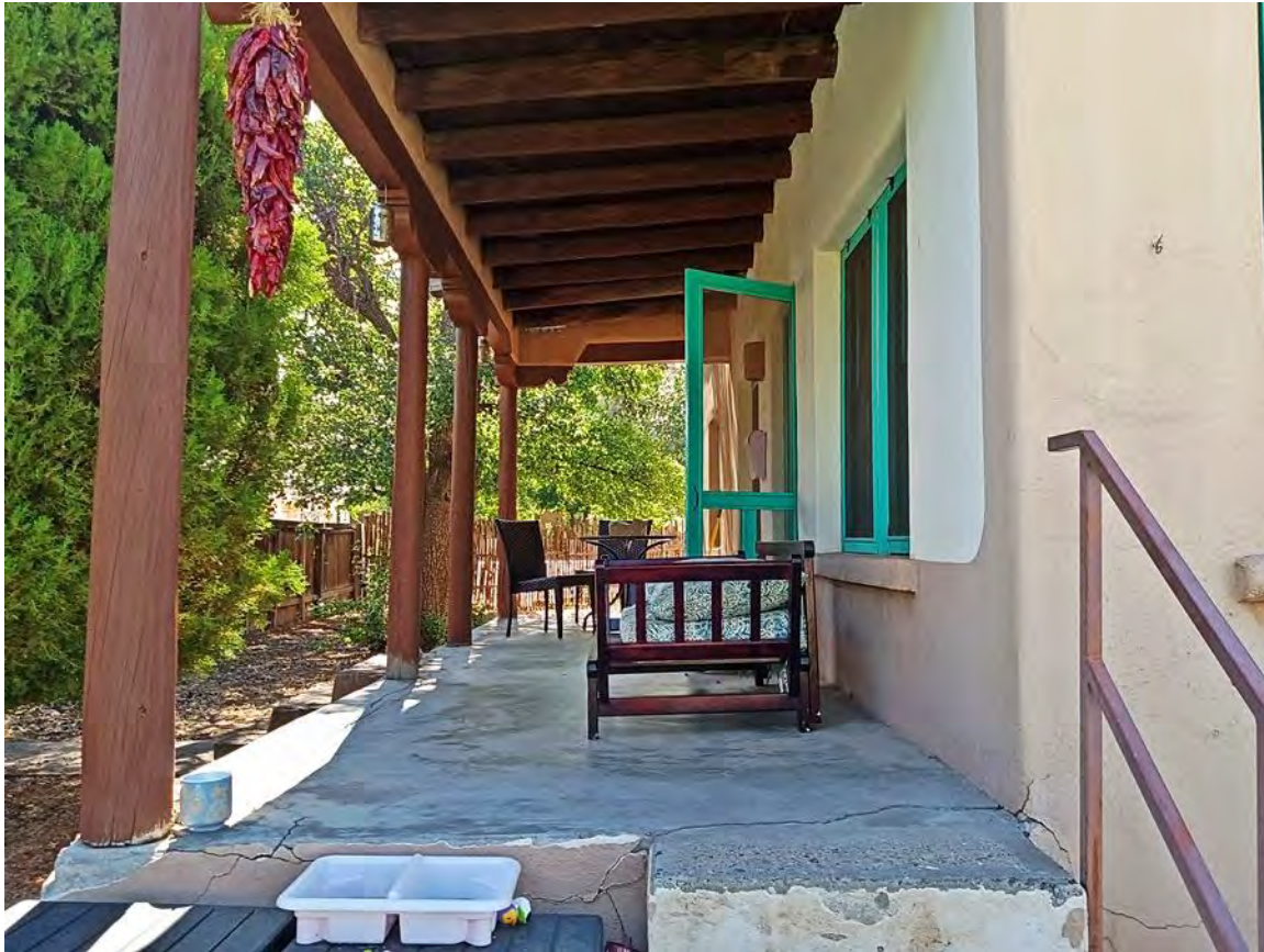
Photo 4: Portal. Camera facing east.
