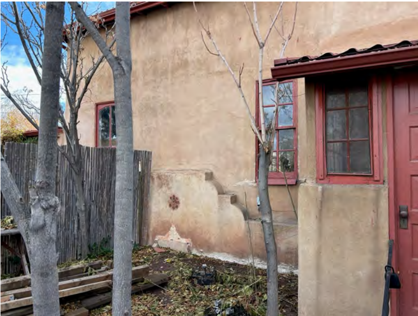
North Elevation - northeast corner of house - thickened wall at exterior with decorative tile and broken spigot (remnants of a fountain)
