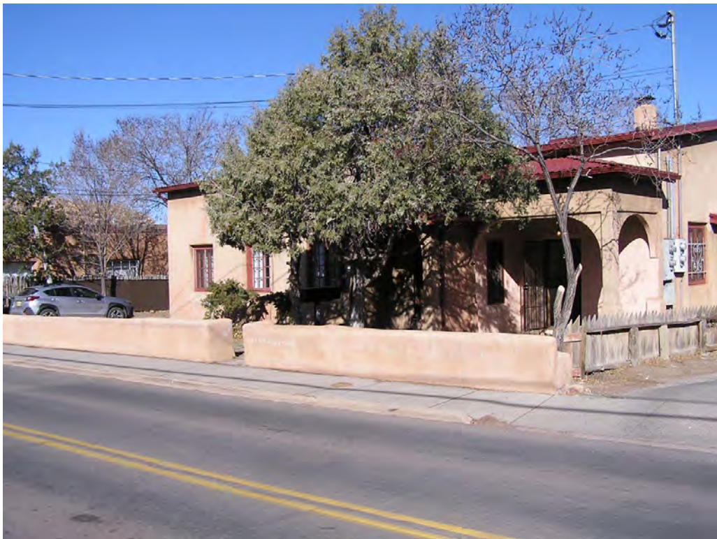
4 - South Façade (facing Agua Fria)
