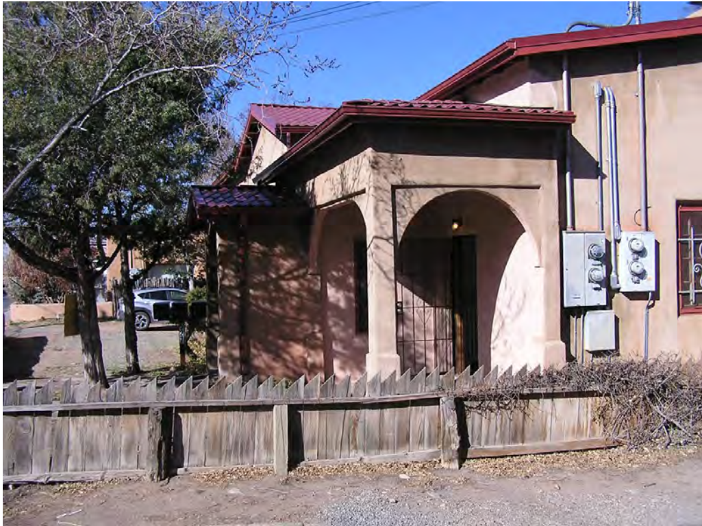
5 - East Façade (southeast corner)
