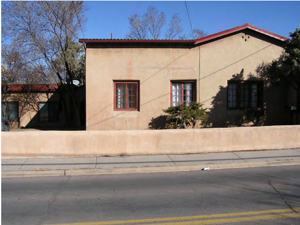
3 - South Façade (facing Agua Fria)
