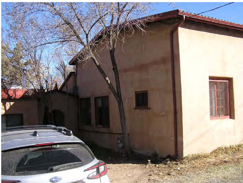
2 - South Façade showing west face of structure
