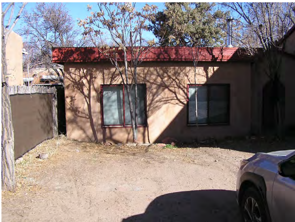
1 - South Façade (facing Agua Fria)
