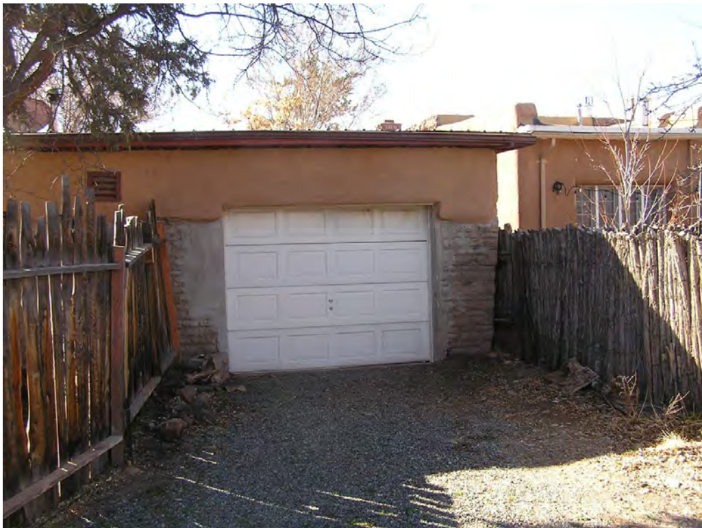
12 - North Façade (northwest corner)
