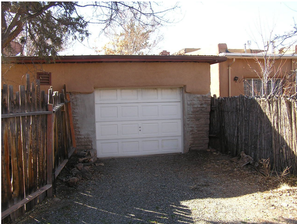
Existing Garage – north façade showing existing garage door
