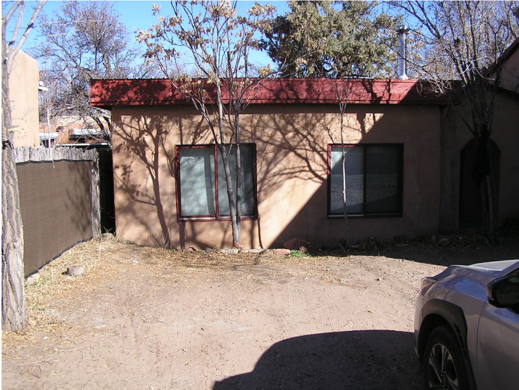
South Façade – Western end of south facing garage structure
