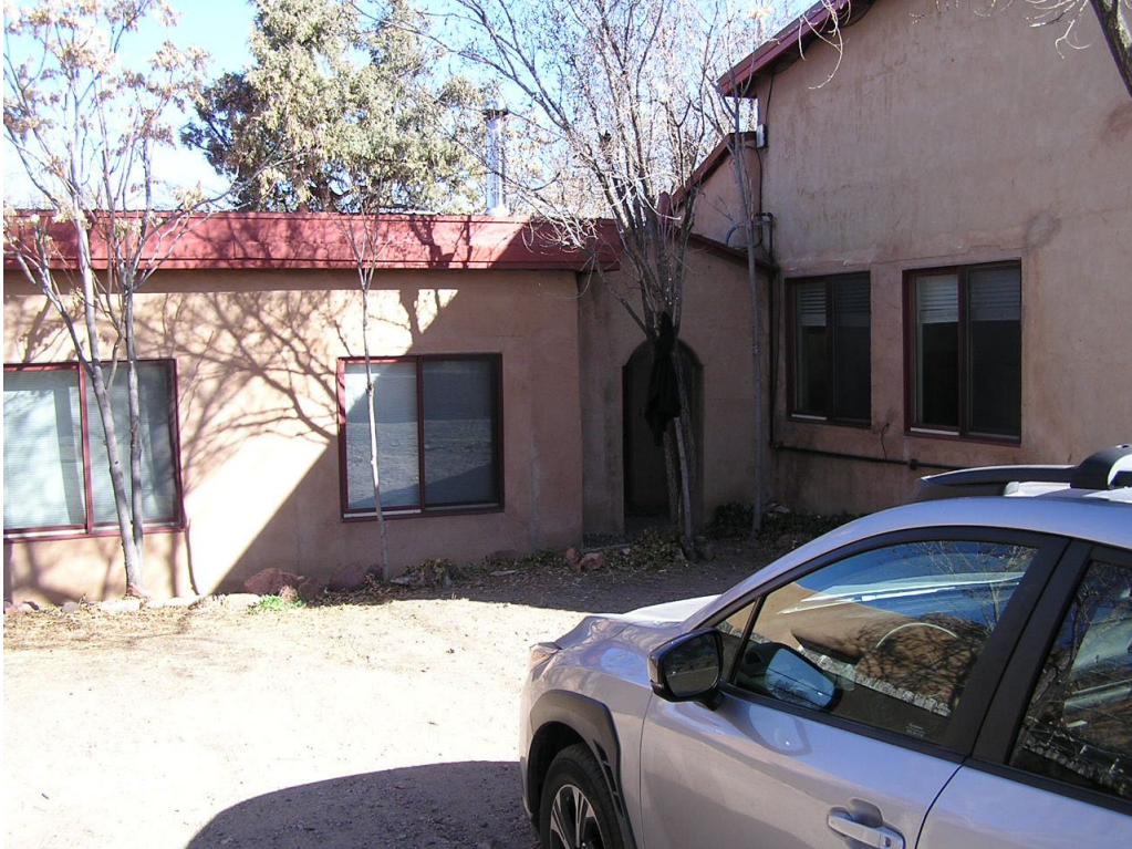
South Façade – Eastern end of south facing garage structure
