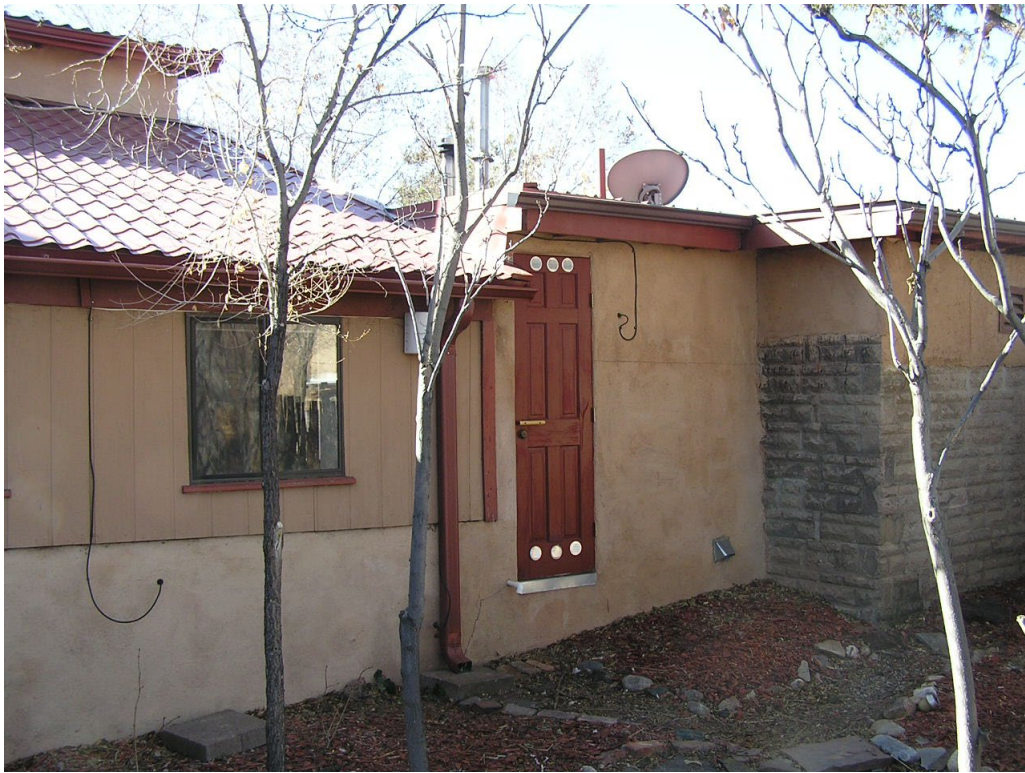
Existing Garage – northeast corner
