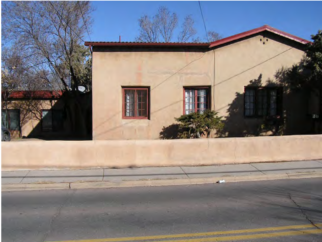
3 - South Façade (facing Agua Fria)
