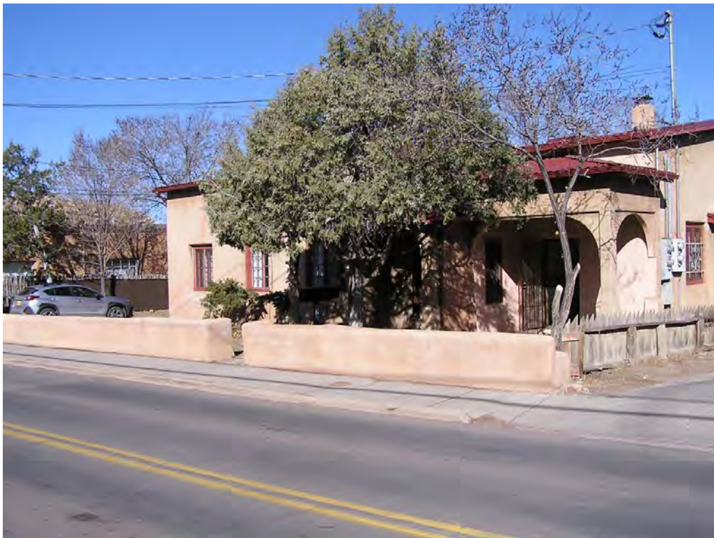
4 - South Façade (facing Agua Fria)
