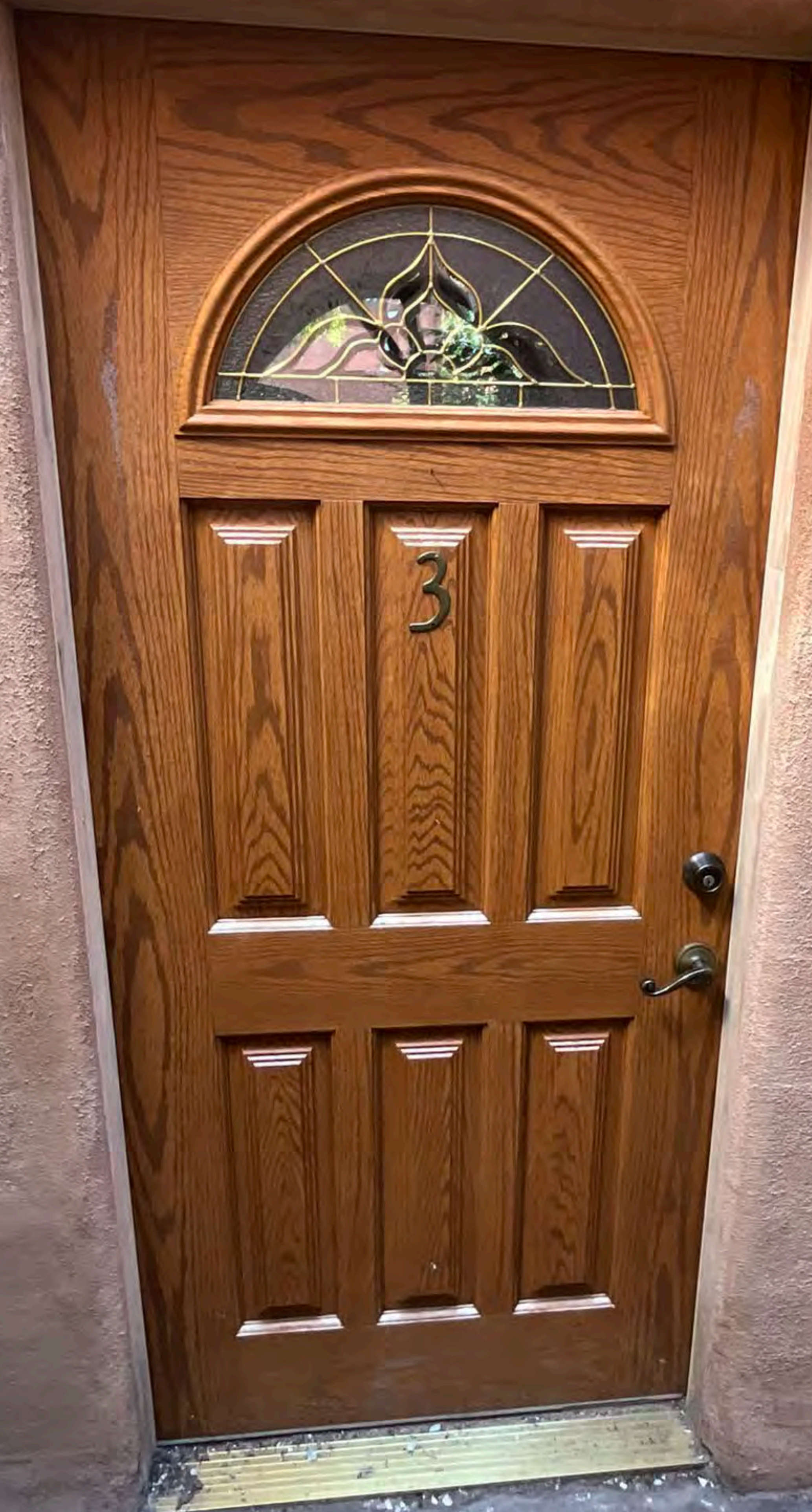
South Elevation Door #1
