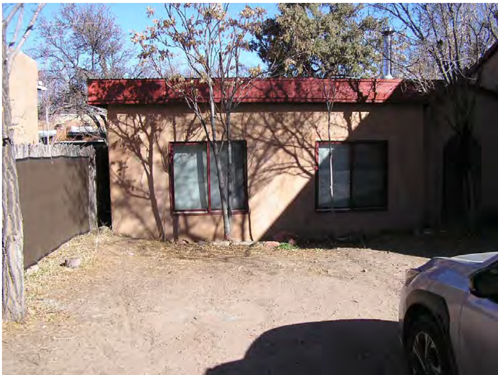
1 - South Façade (facing Agua Fria)
