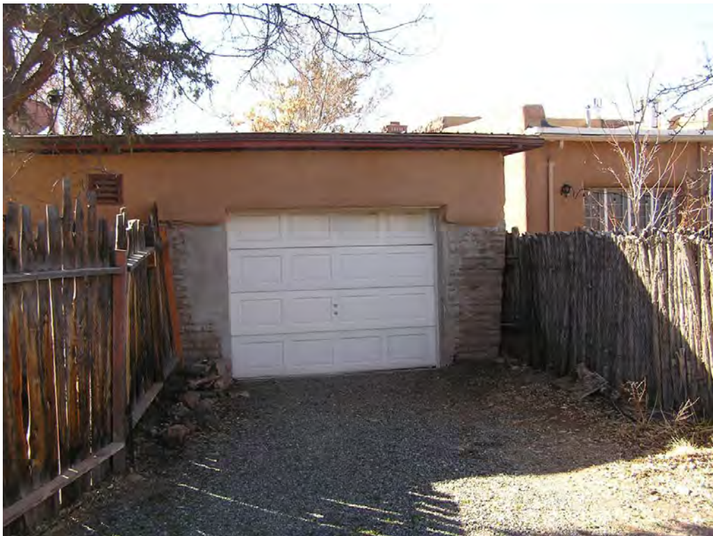
12 - North Façade (northwest corner)
