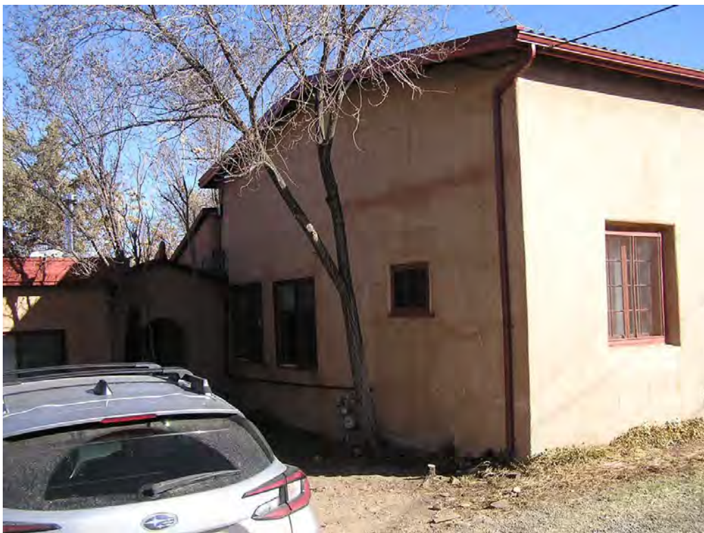
2 - South Façade showing west face of structure
