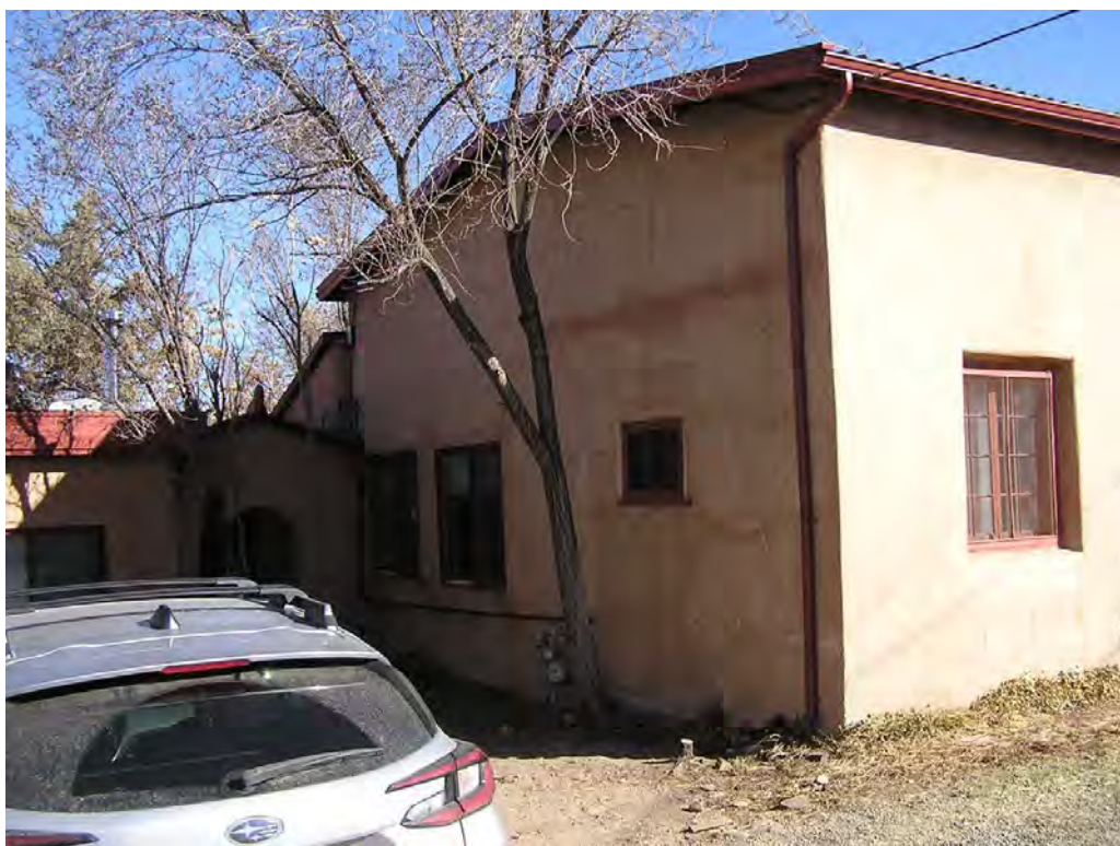
2 - South Façade showing west face of structure
