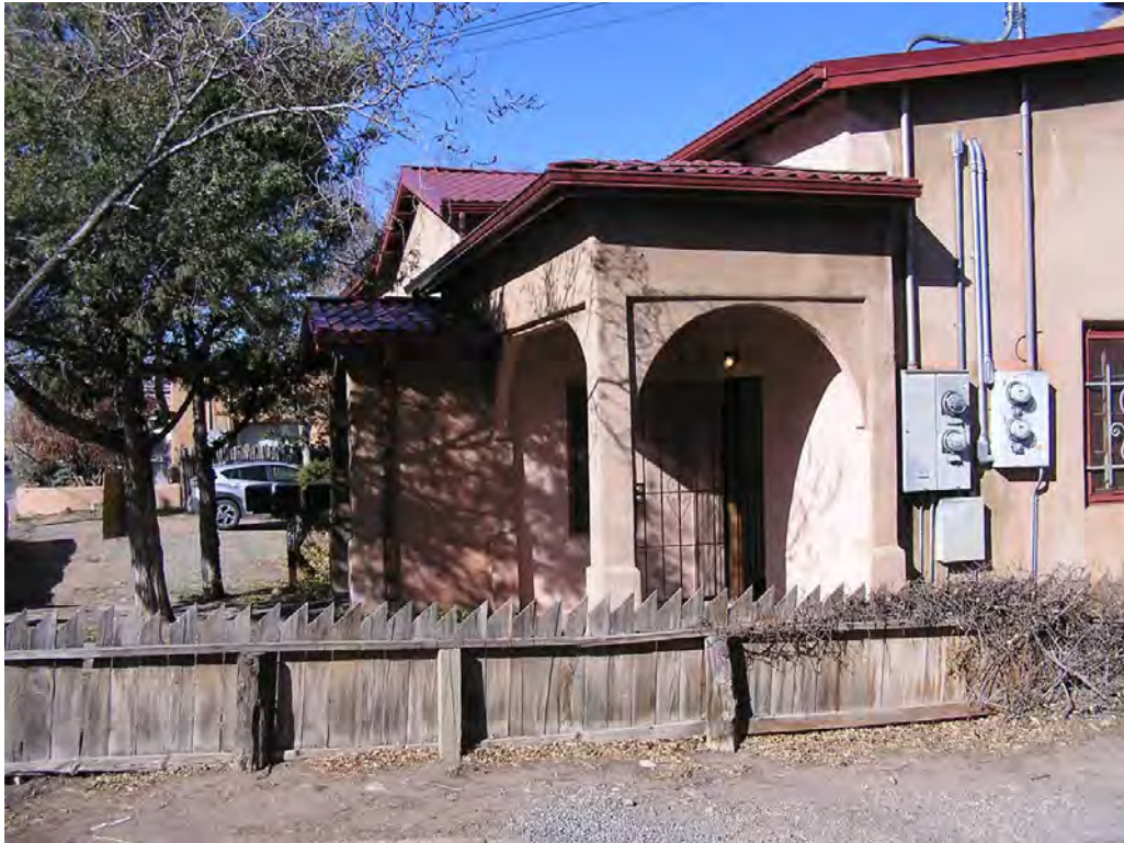
5 - East Façade (southeast corner)
