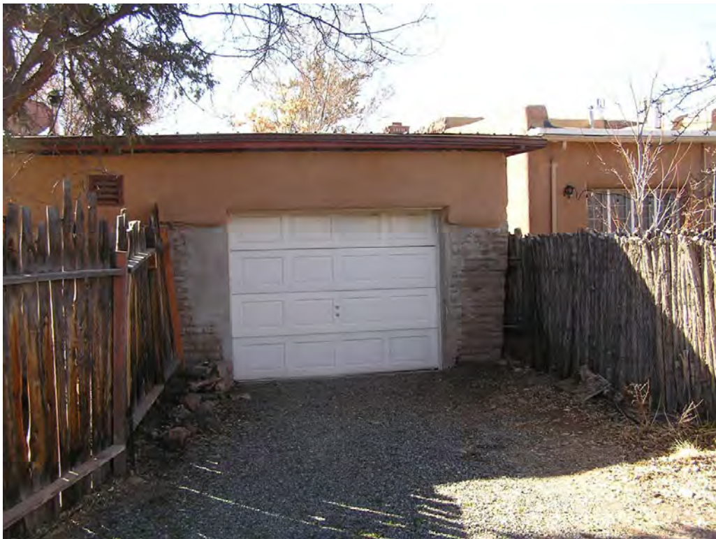
12 - North Façade (northwest corner)
