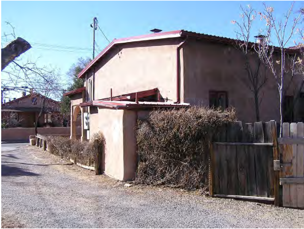
7 - North Façade (northeast corner)
