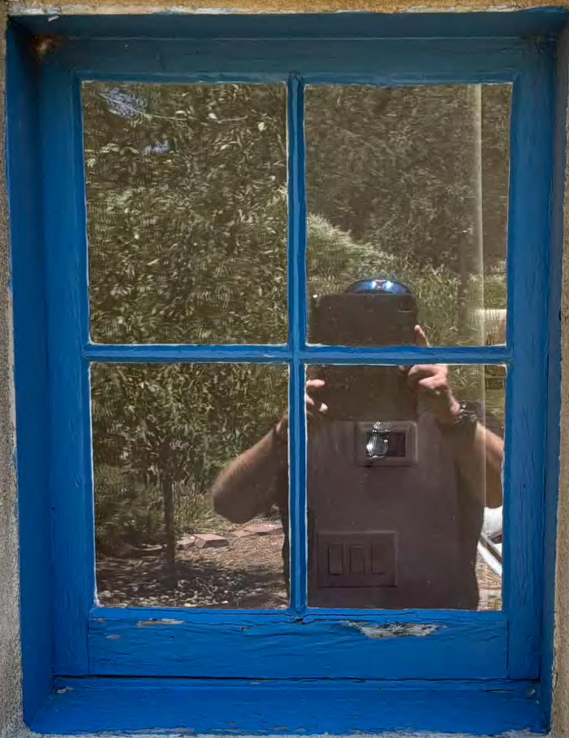
North Elevation Casita Window C-B.
