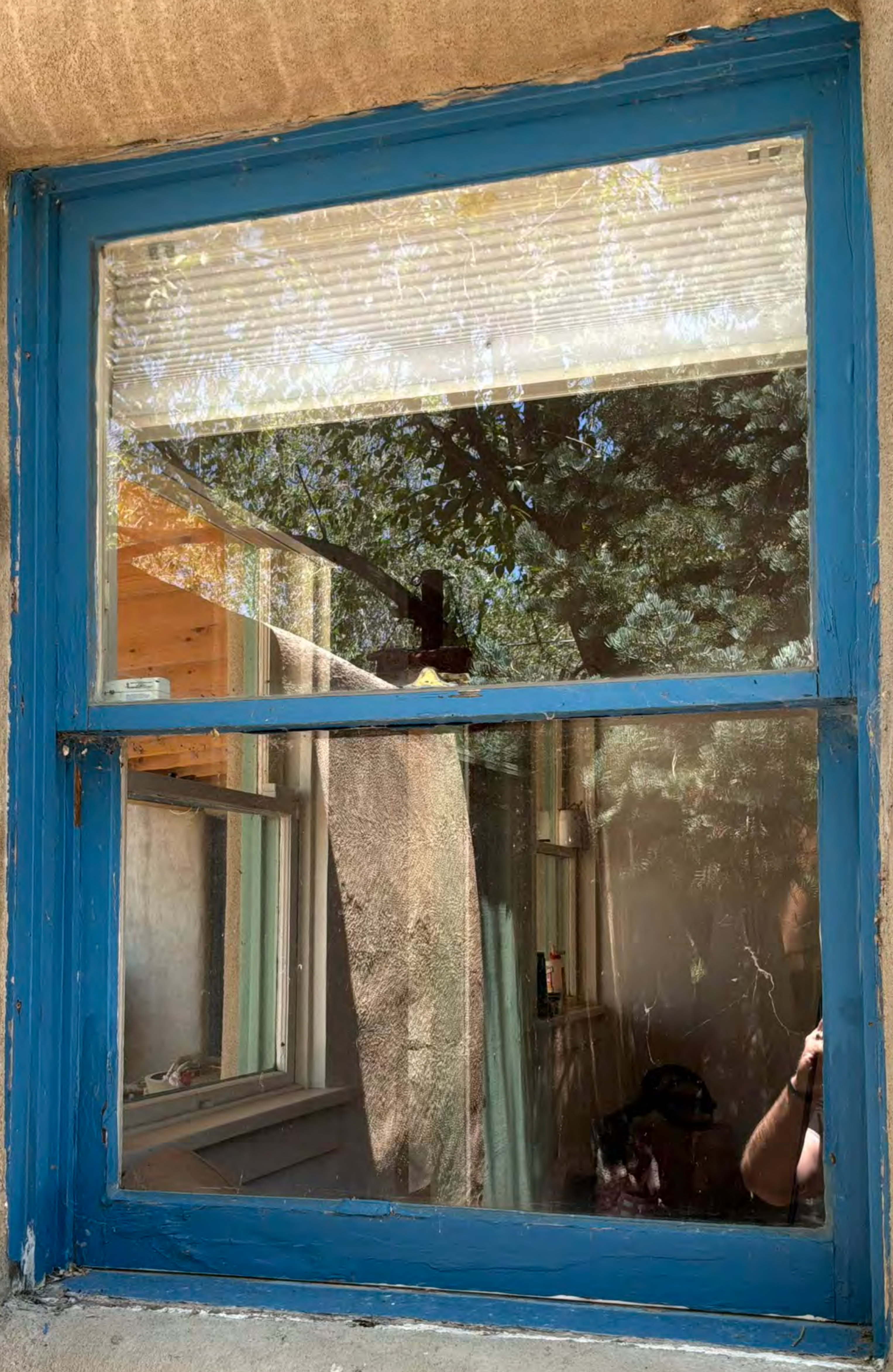
North Elevation Window I.
