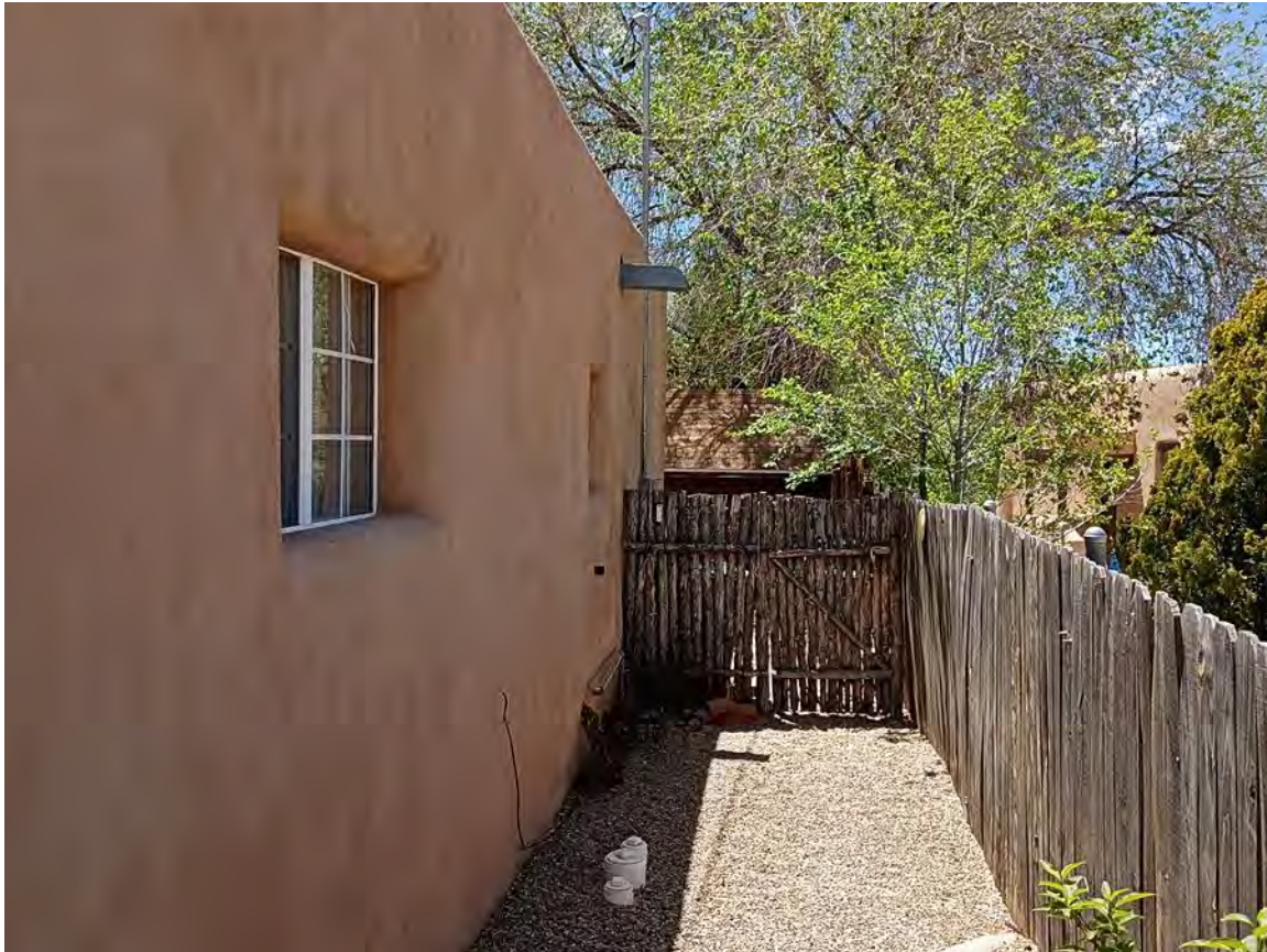
Photo 7: North elevation. Camera facing west.
