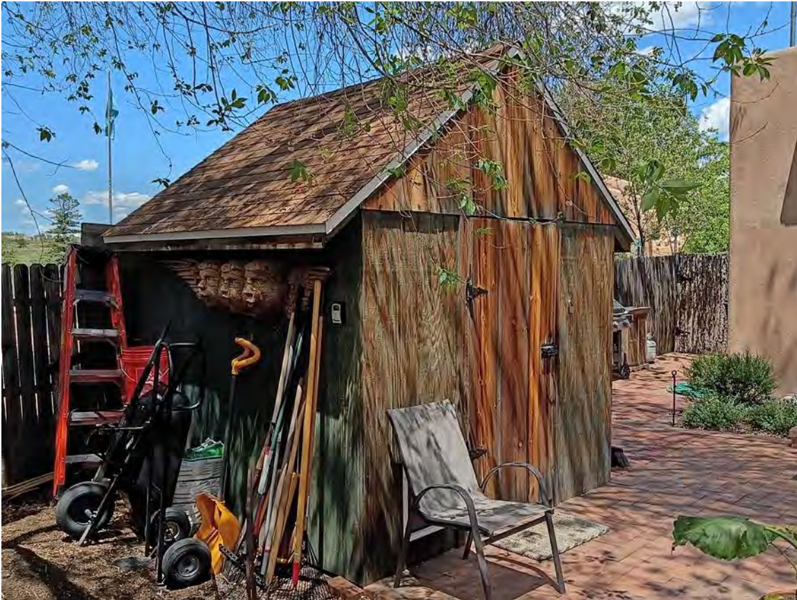
Photo 14: Shed. Camera facing northeast.
