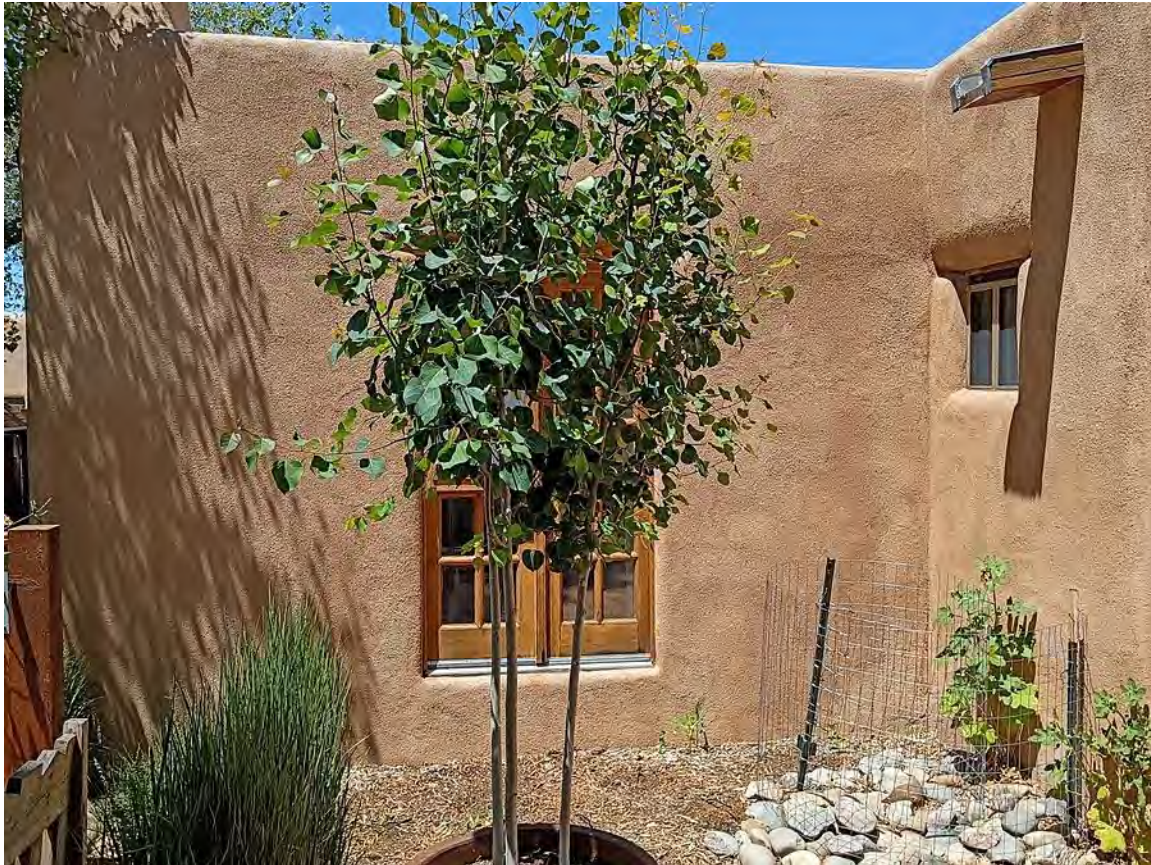
Photo 5: South elevation, west end. Camera facing north.
