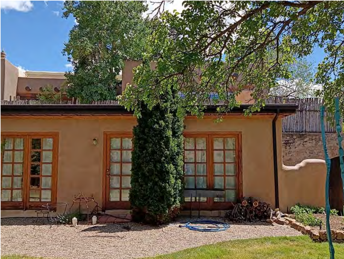
Photo 11: North elevation, west end. Camera facing south.
