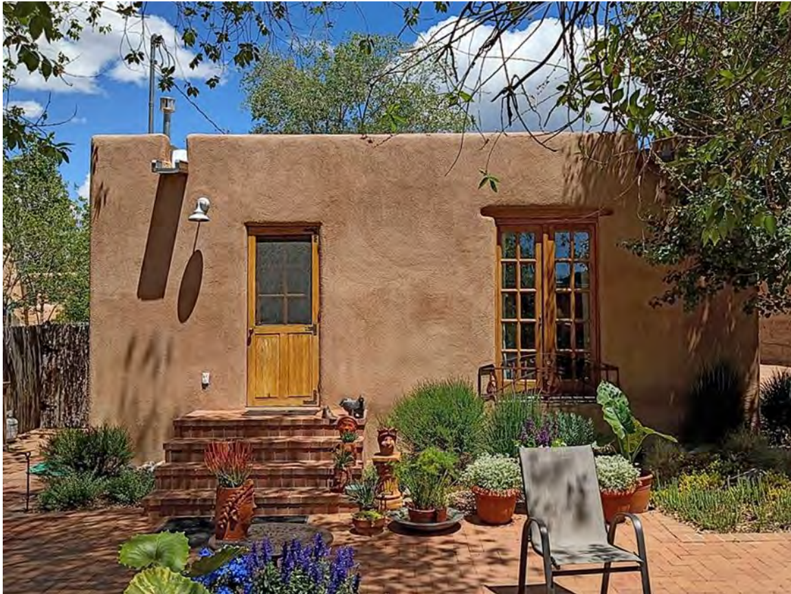
Photo 6: West elevation. Camera facing east.
