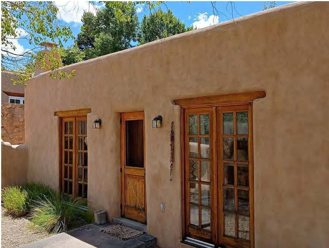
Photo 3: East (front) façade. Camera facing southeast.
