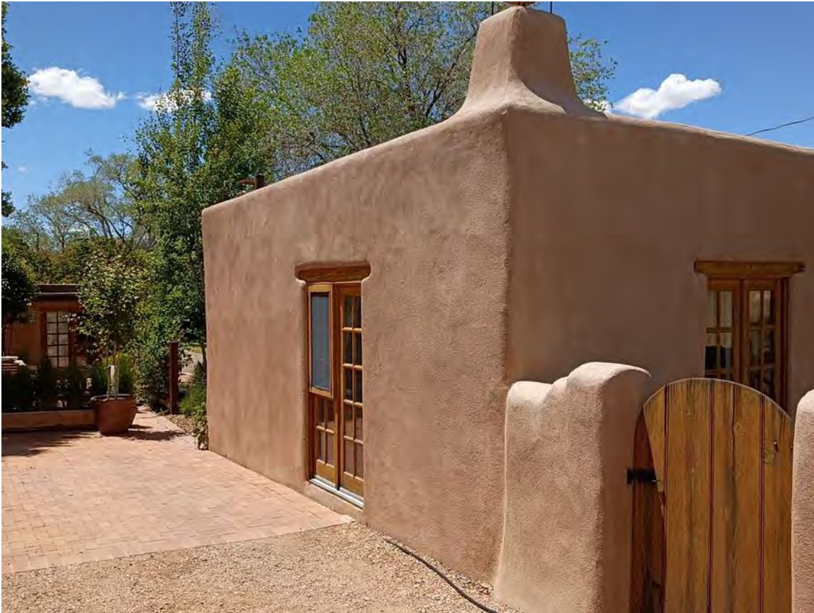
Photo 4: South elevation, east end. Camera facing northwest.
