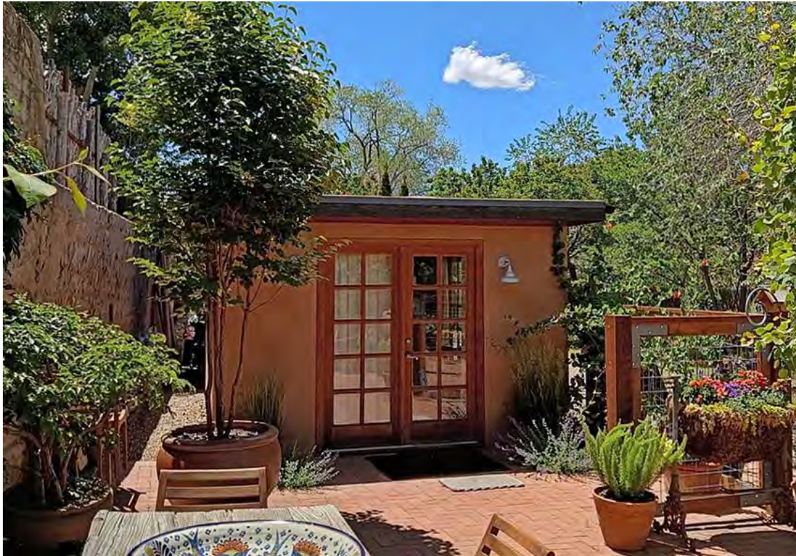
Photo 9: East (front) elevation. Camera facing northwest.
