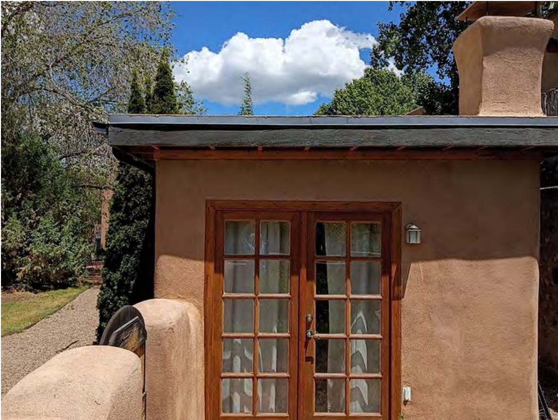
Photo 12: West elevation. Camera facing east.
