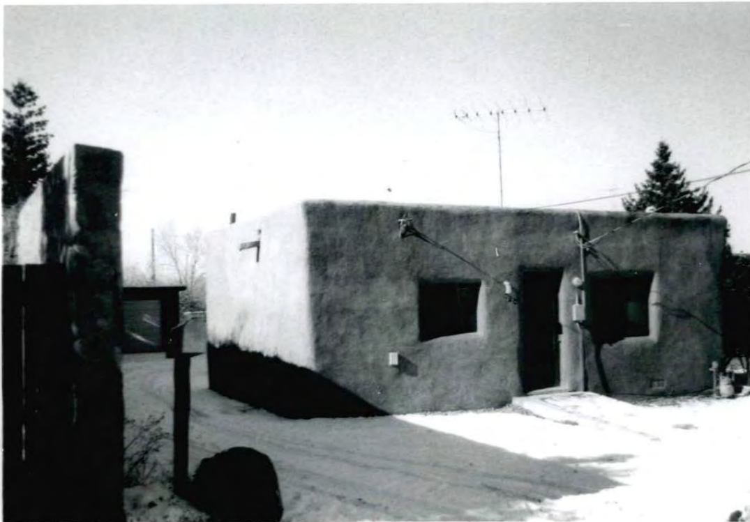
Figure 1: October 30, 1984, Historic Building Inventory form photograph. East (front) and south elevations, looking northwest. Michael Belshaw.
