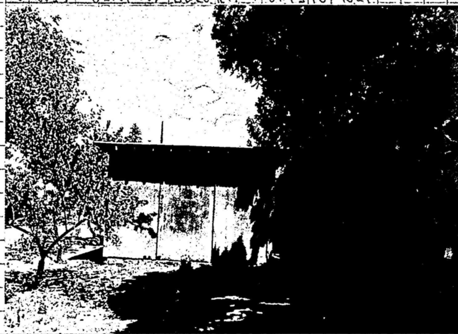
GARAGE: WEST FACADE
