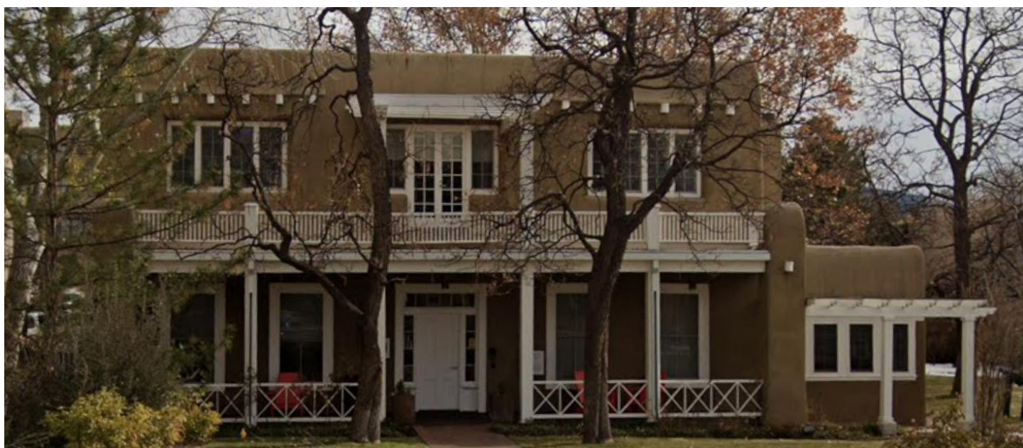
Figure 3: The west elevation showing the porch, pergola, and trellis structures.
