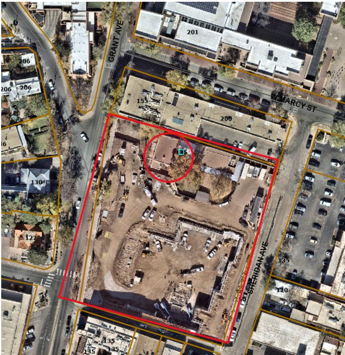
Figure 1: Property Location with Subject Building Circled
