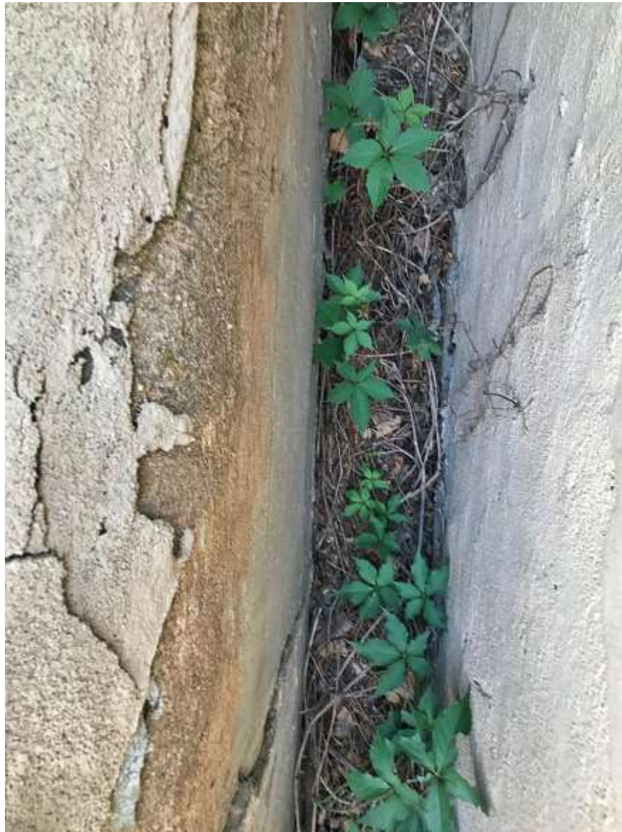
Figure 9: "East Section," south elevation, left, Safeway Building, right. July 2, 2023, John W. Murphey.
