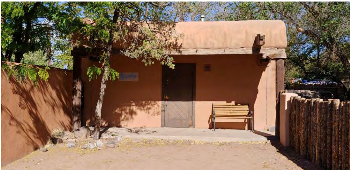
Photo 8: Studio, west (front) elevation. Camera facing east.
