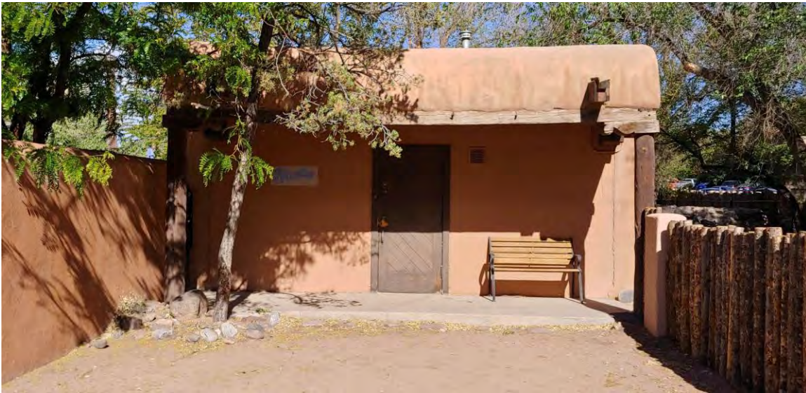
Photo 8: Studio, west (front) elevation. Camera facing east.
