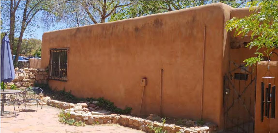
Photo 9: Studio, north elevation Camera facing southeast.
