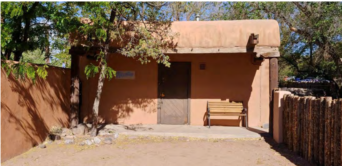
Photo 8: Studio, west (front) elevation. Camera facing east.
