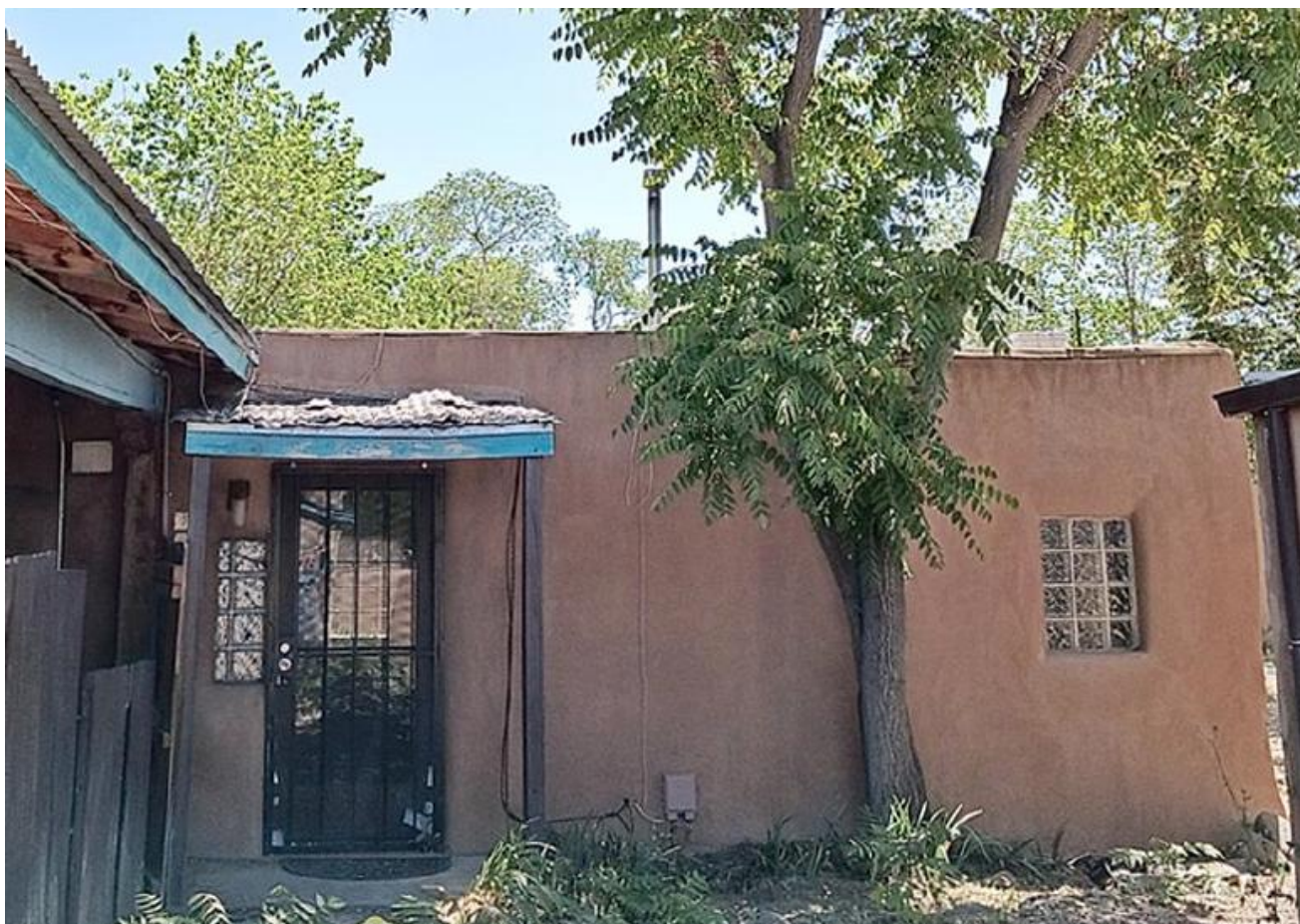
Figure 5. 405 Juanita Street, Unit B, west elevation. Source: September 2, 2026, HCPI, John W. Murphy, photographed by Jim Rodman May 19, 2026.
