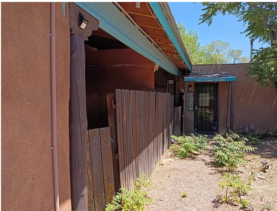
Photo 5: South elevation, east end. Nonfunctional carports, left; altered fenestration of earlier apartment, center. Camera facing east.
