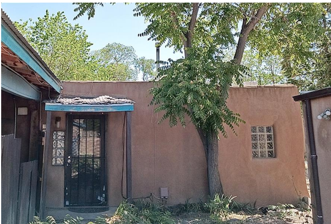
Photo 7: West elevation, south end. Camera facing east.
