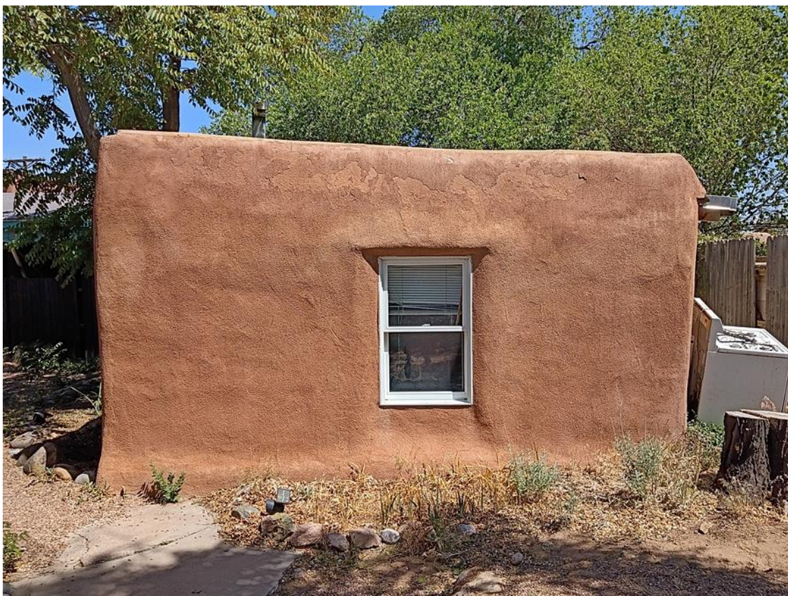
Photo 8: South elevation. Camera facing north.
