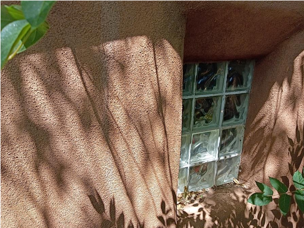
Photo 10: East elevation opening infilled with glass block. Camera facing down.
