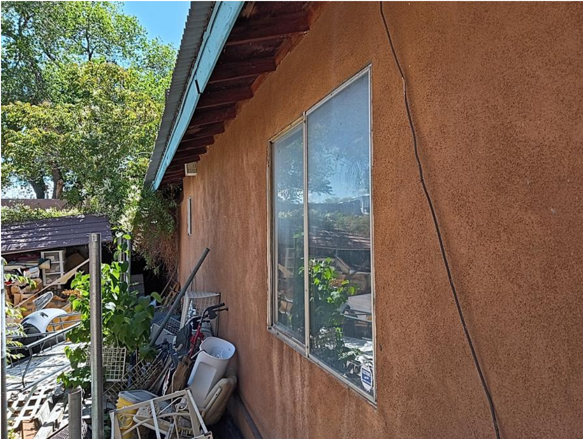
Photo 6: North elevation. Camera facing southeast.
