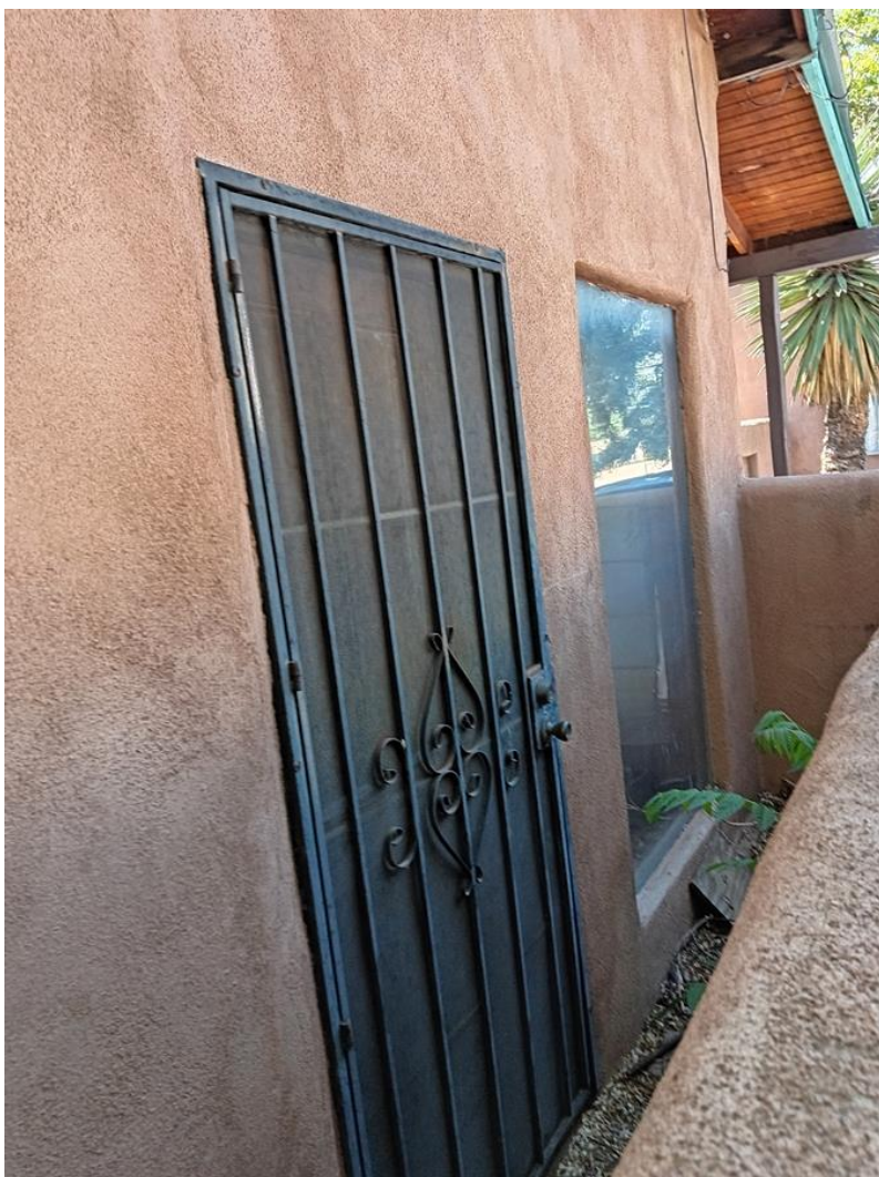
Photo 3: West (front) elevation. Fenestration of non-historic infill of carport. Camera facing southeast.
