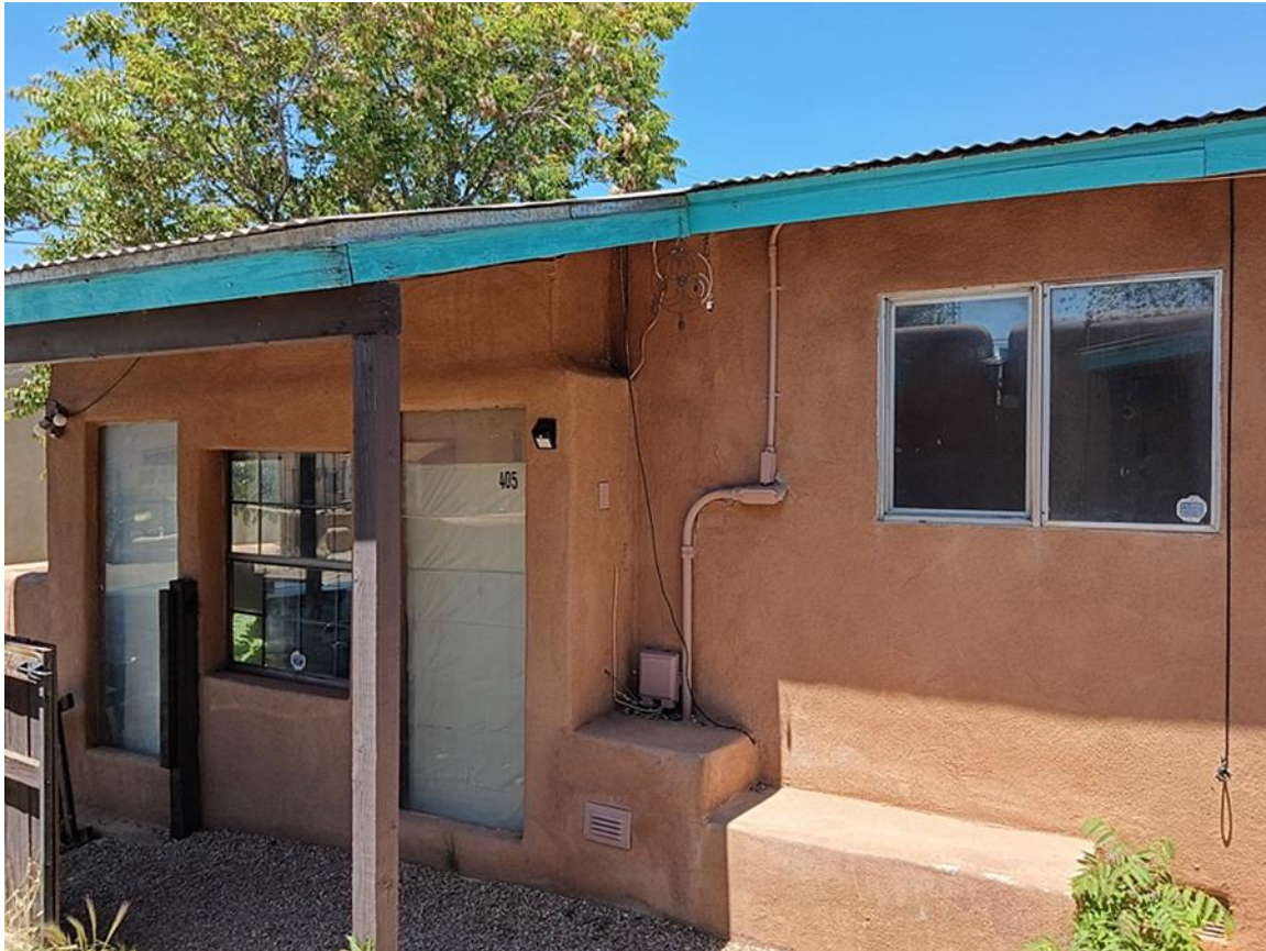
Photo 4: South elevation, west end. Non-historic infill of carport at right. Camera facing northwest.
