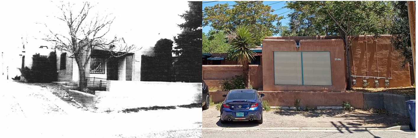
Figure 7. 407 Juanita Street west elevation. Source: HCPI August 1985 (left); HCPI September 2, 2026 (right).
