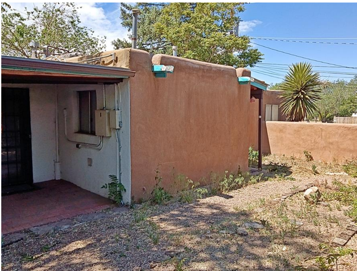
Photo 6: North elevation, post-1958 addition, west end. Camera facing southwest.
