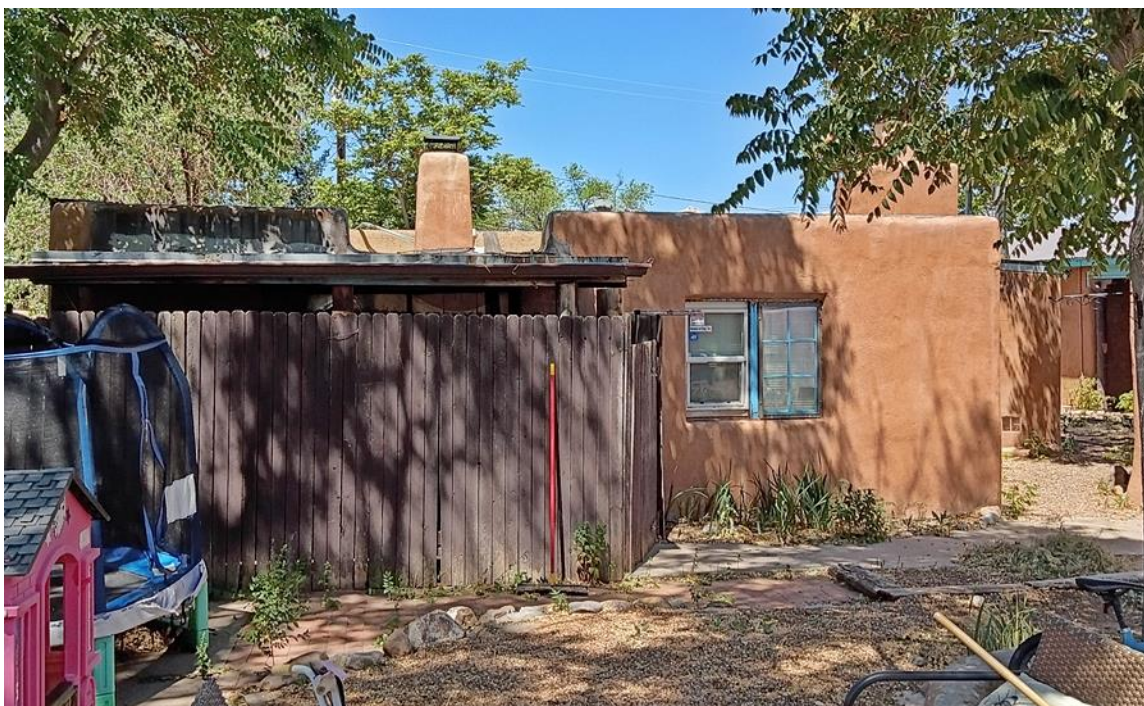
Photo 9: East elevation. Area behind fence not visible. Camera facing west.
