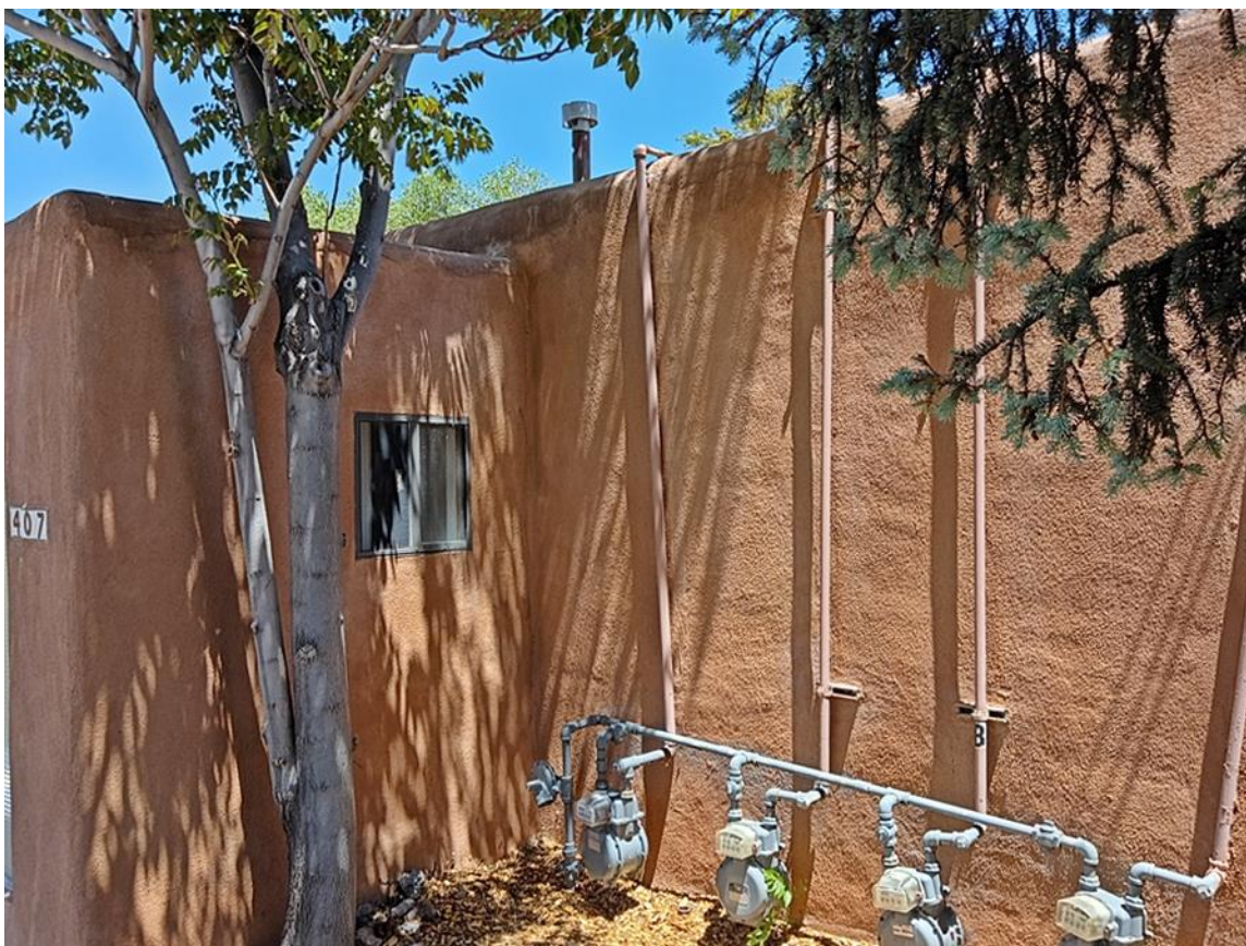
Photo 3: West (front) elevation, south side. Enclosed portal at left. Camera facing northeast.
