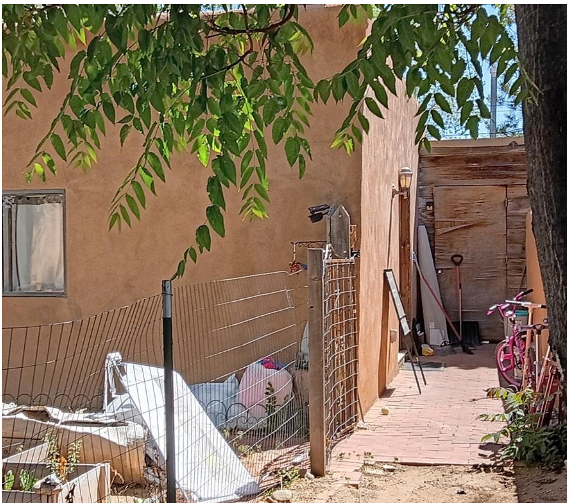
Photo 14: South elevation. Camera facing east.
