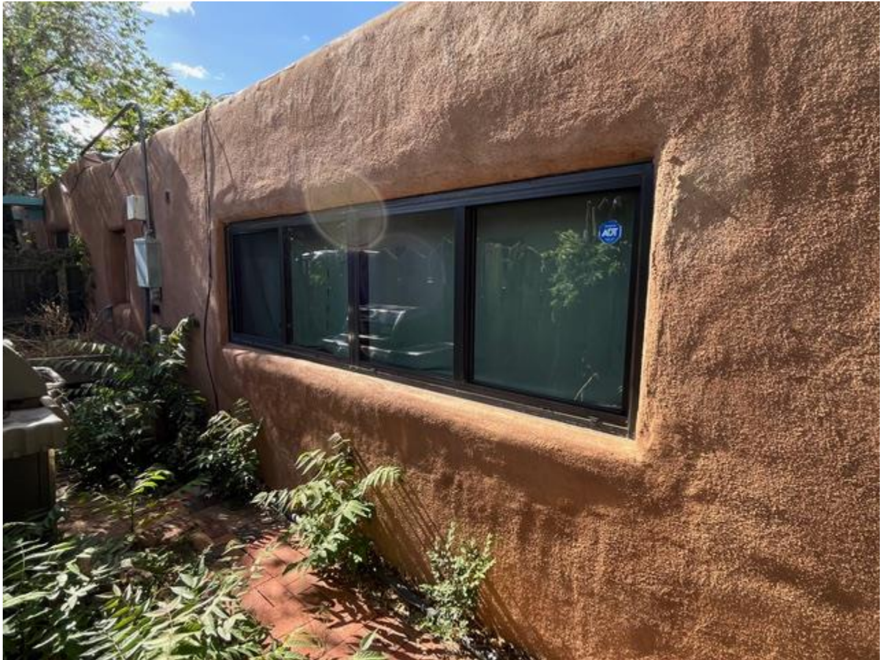
Photo 12A: South elevation. Camera facing northwest. May 2026, Antoine el-Khoury.
