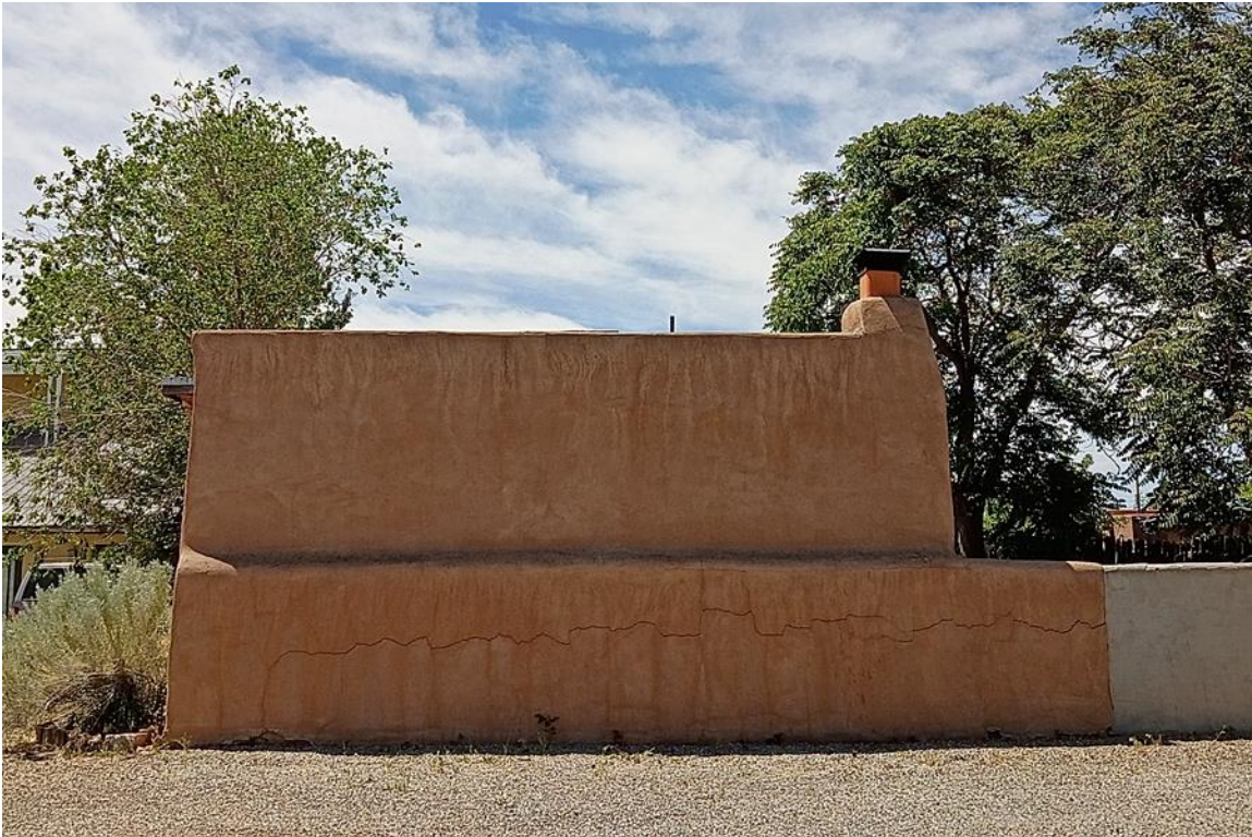
Photo 15: North elevation. Camera facing south.
