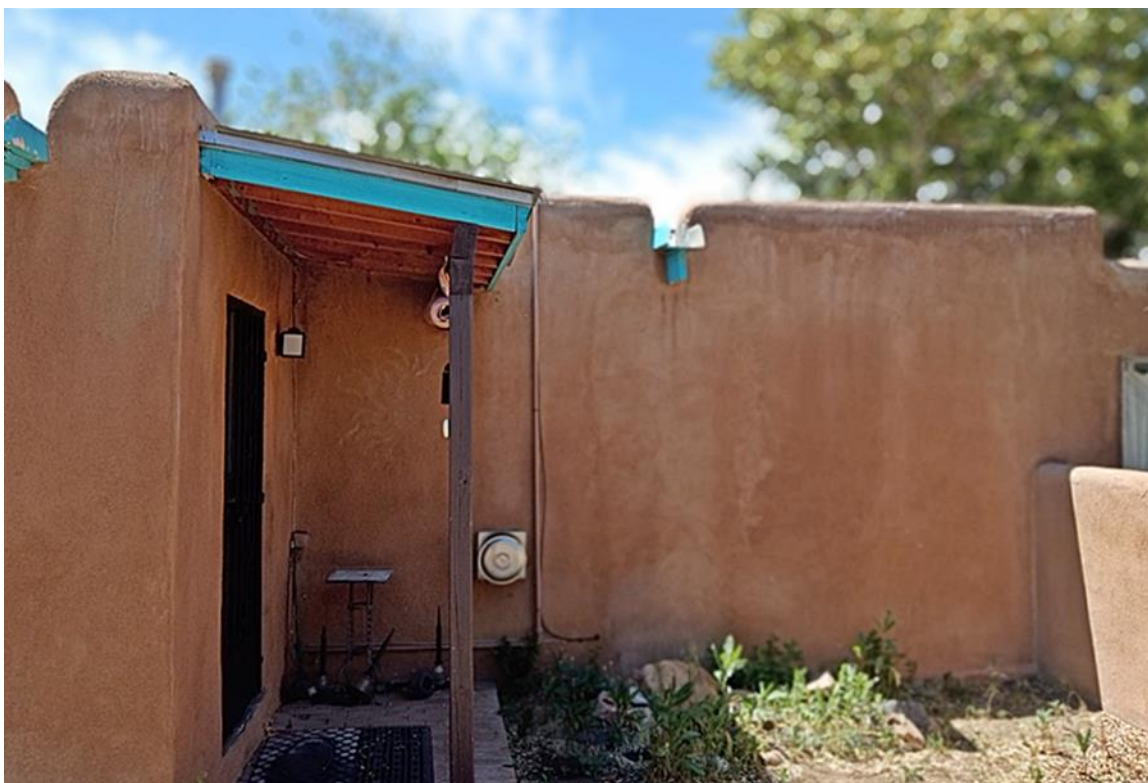
Photo 4: North elevation, west end. Location of new entry at left; removed window at right. Camera facing south.
