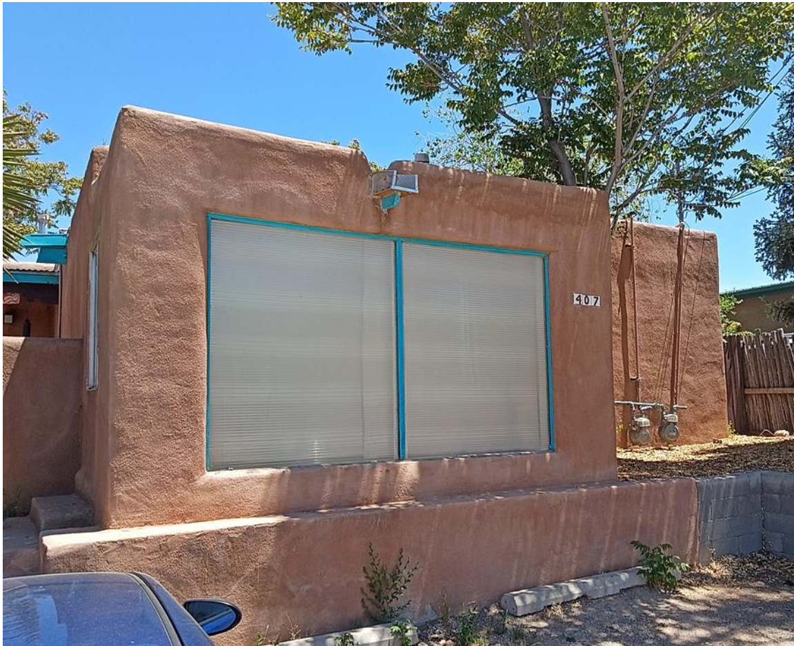
Photo 2: West (front) elevation, north side. Non-historic enclosure and modification of portal. Camera facing Southeast.
