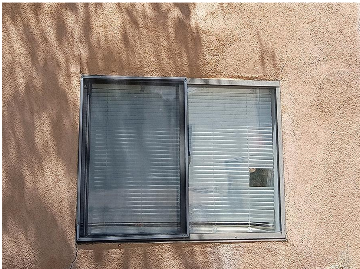
Photo 17: East elevation. Window detail. Camera facing west.
