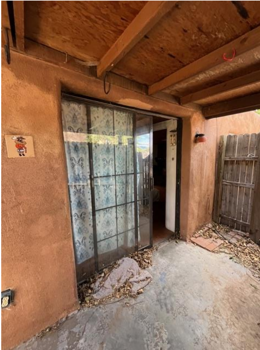
Photo 9A: East elevation. Camera facing northwest. May 2026, Antoine el-Khoury.
