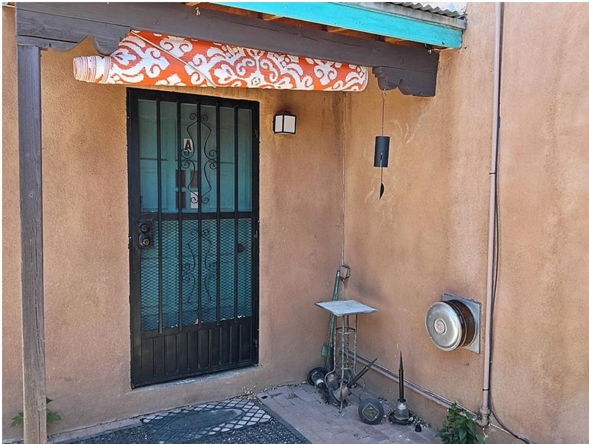
Photo 5: West elevation. Non-historic entry and porch. Camera facing southeast.
