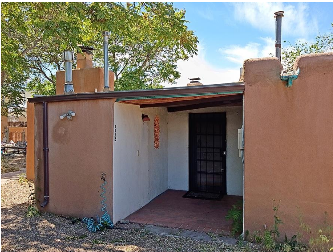
Photo 7: North elevation, post-1958 addition, east end. Camera facing southeast.
