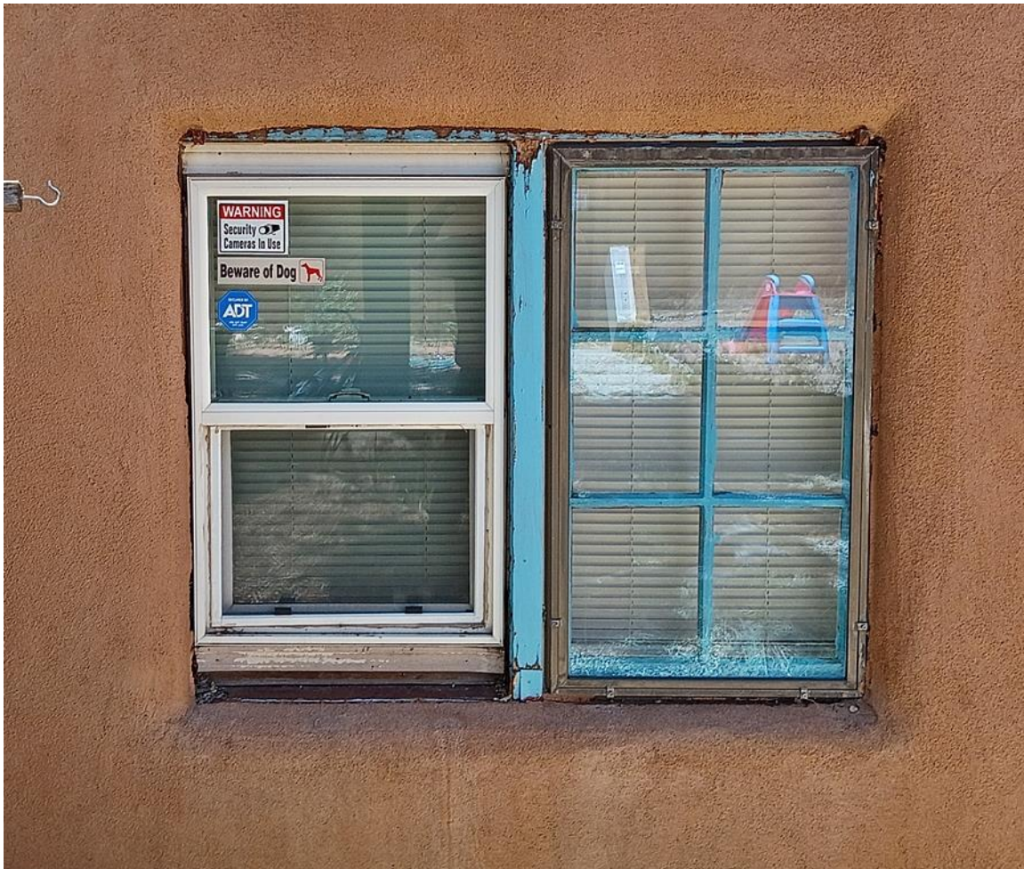
Photo 10: East elevation. Window detail. Camera facing west.
