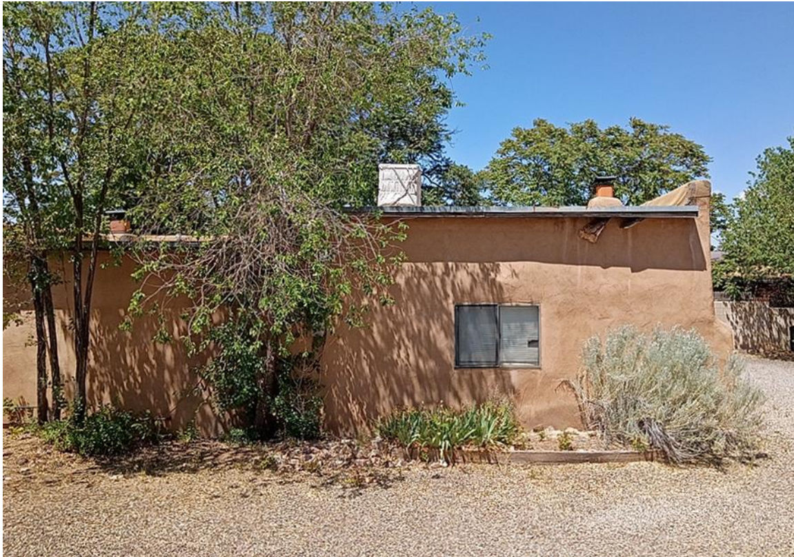
Photo 16: East elevation. Camera facing west.
