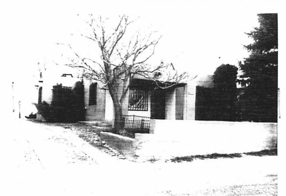
Figure 10: August 1985 HBI survey photograph showing original design, including entry portal and different front wall. Creator: Harry Weiss.
